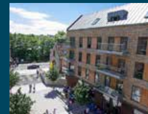
Wapping Wharf, Bristol 200 dw/ha
