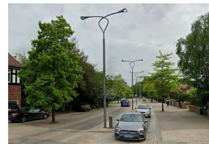
Signature lighting columns and perceptual narrowing of the carriageway through a central median(Poynton, UK)
