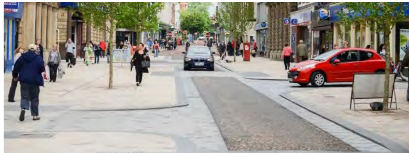
Visually narrowed carriageway
