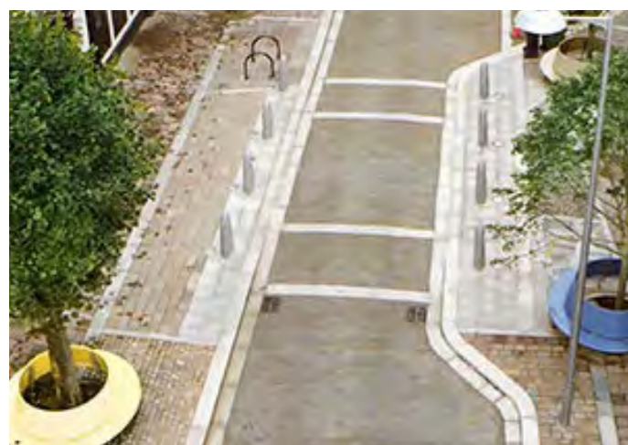
Pinch points and defensive street furniture (Cockermouth, UK)
