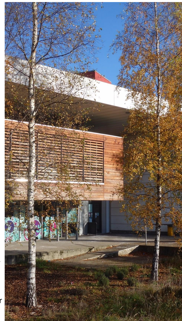
Fig 4.a.3 The Bridge, Easterhouse’s civic heart.
