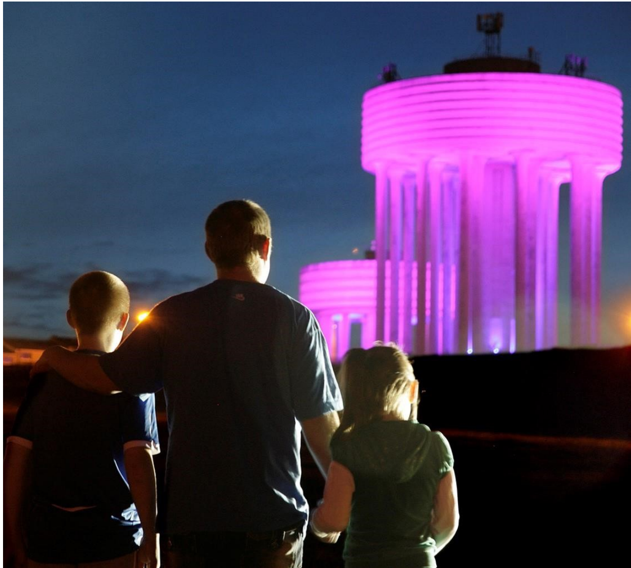
Fig 4.b.2 - A family watching the illumination of the Garthamlock Water Towers.
