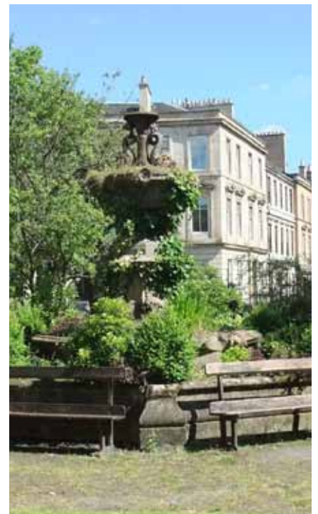
1 Detail of roofscape St Georges Mansions, Burnet and Boston , 1902, Woodlands Rd - St Georges Rd/ 2 Communal Gardens, Queens Cres
