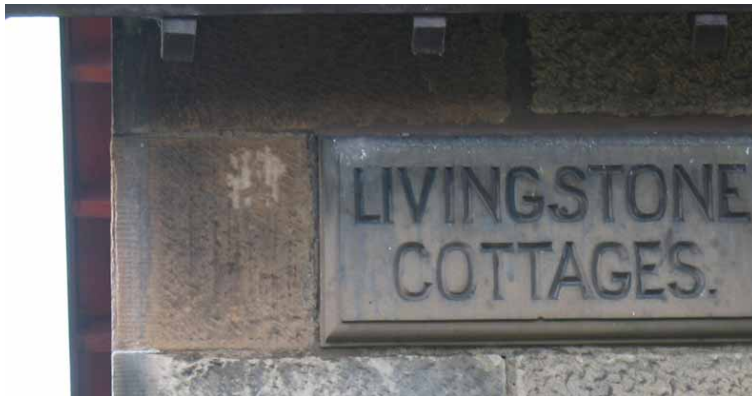
1 Example of notable feature of the area - Names of groups of cottages carved into the stone of the dwellings. Livingstone Cottages, Victoria Park Street
