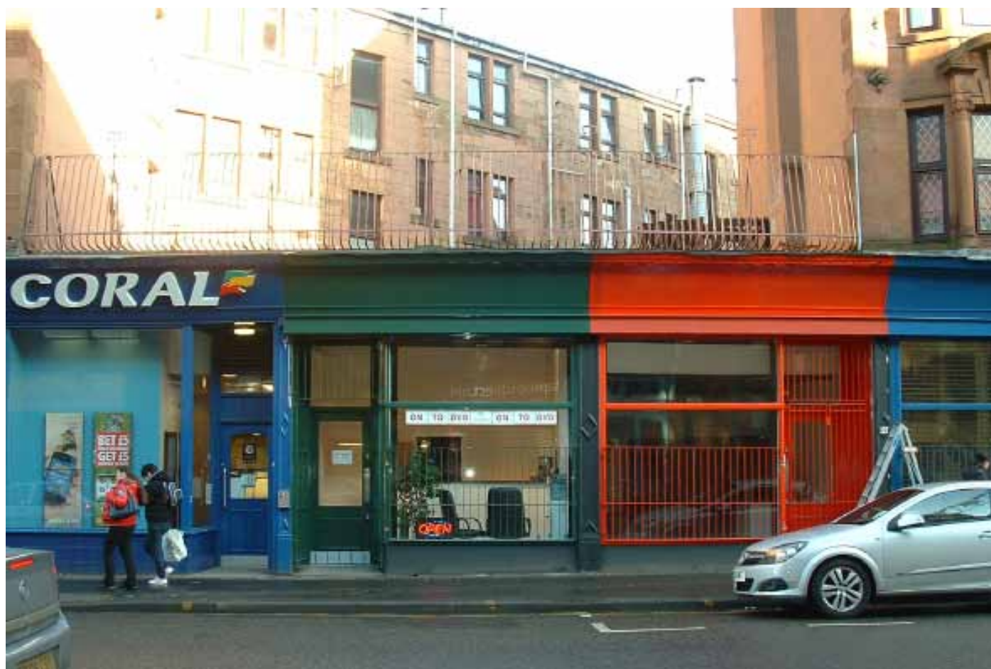
1 Example of restoration to shopfronts
