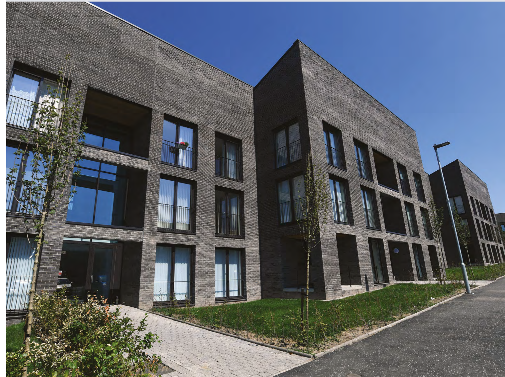
Dunira Street (Tollcross Housing Association)
