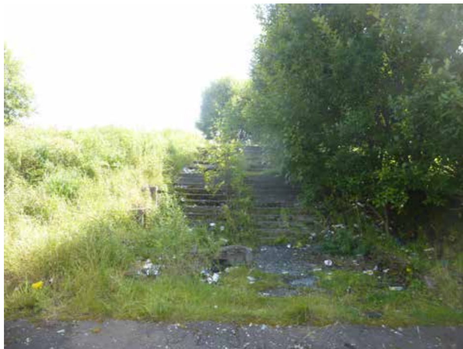
4. DERELICT STEPS TO SOUTH OF SITE
