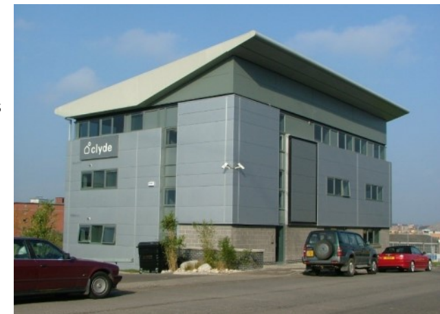
Fig 4a.2 - Craighall Business Park - office units in an accessible location.
