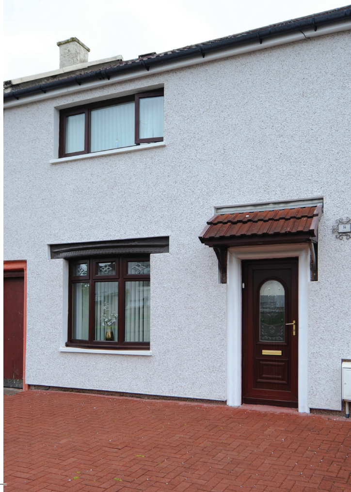
Before & After External Wall Insulation, Milton
