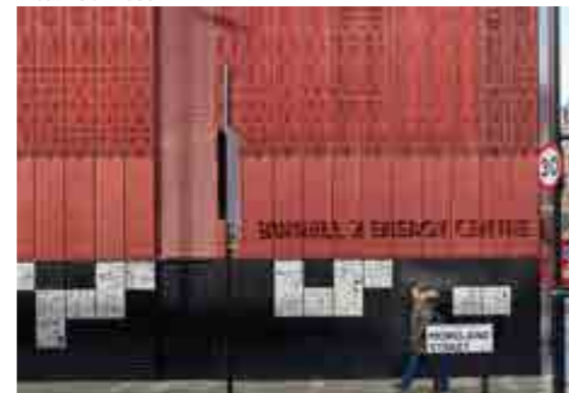
Bunhill Energy Centre - Cullinhanstudio.com
