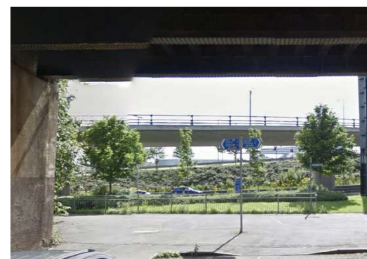
The A814 Clydeside Expressway as a barrier to connectivity.
