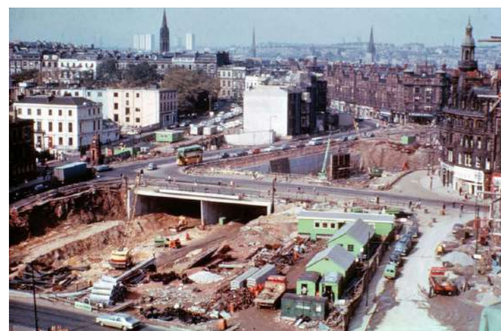
The M8 in construction at Charing Cross in the 1960s.
