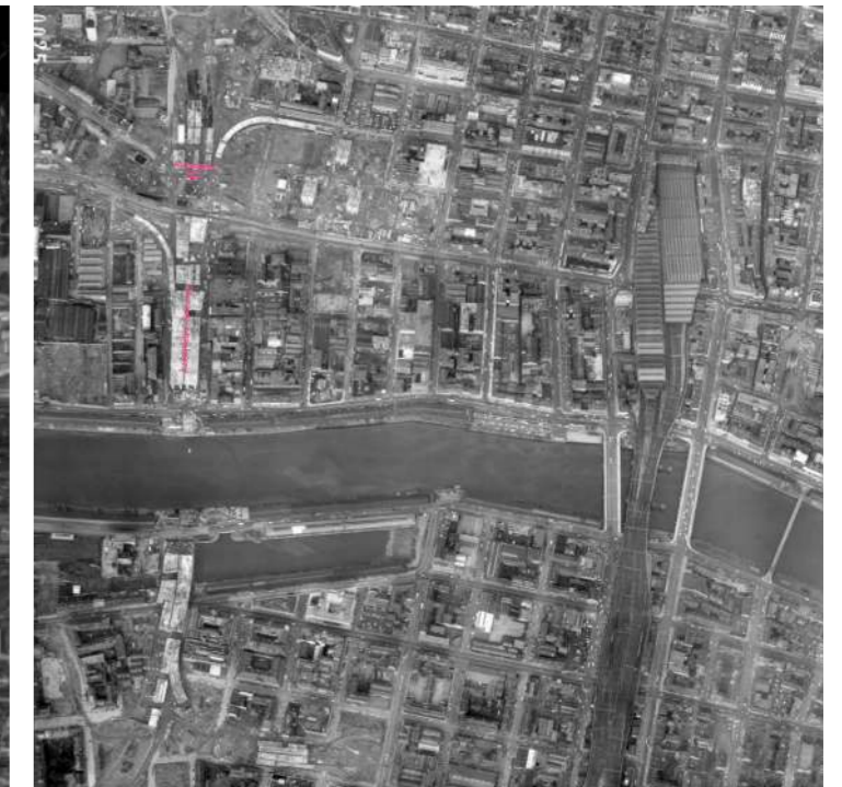
Motorway and Kingston Bridge in Construction
