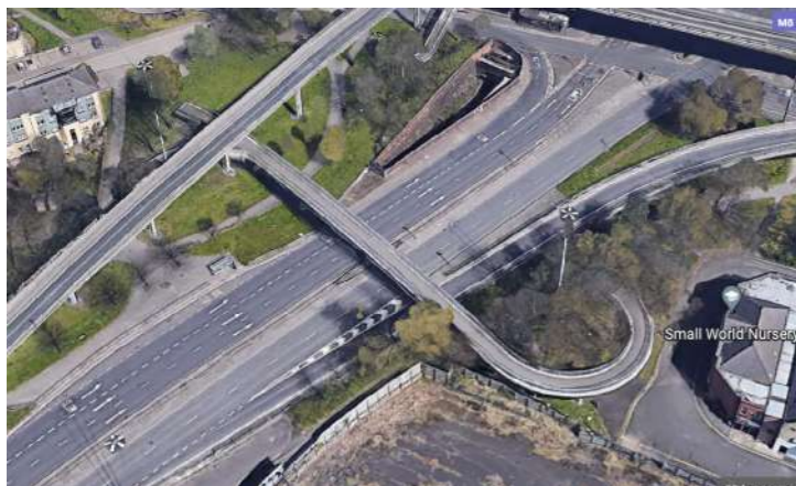
5 - Footbridge connecting Anderston to the Riverfront. To the north, the bridge does not connect well with Argyle Street and the surrounding area. Either side of the connection the bridge creates a series of non-spaces. The same can be said for the area around most of the following footbridges.
