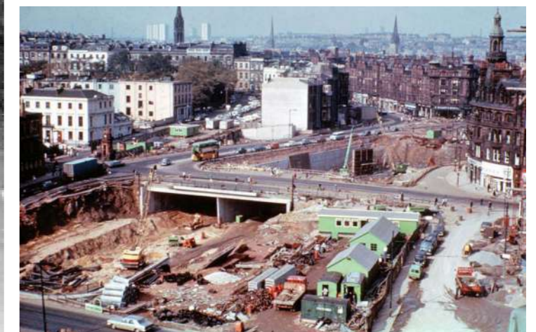
Construction of the M8 at Charing Cross
