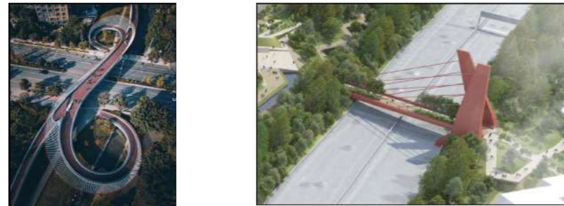
Pedestrian Bridges over Expressways
