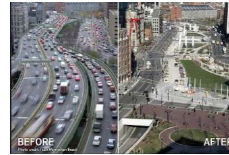
Boston Central Artery Before and After
