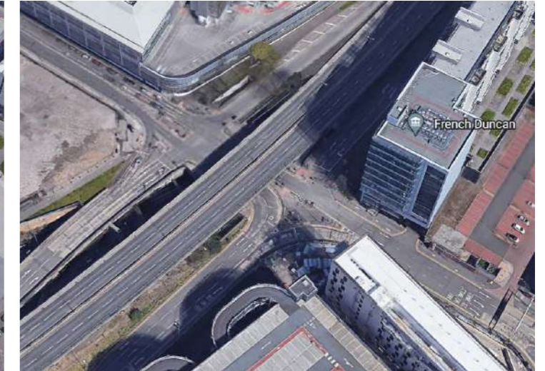
4 - Underpass connecting Finnieston to the Riverfront. The underpass is dark and largely unused. Instead people opt to walk across the road at this junction. Car dominance makes this place very hostile for pedestrians and cyclists.
