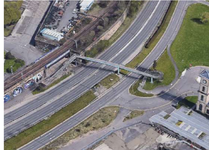
2 - Footbridge between SWG3 Area and River Front at the Clydeside Distillery. Here there is a narrow path which is non DDA compliant. Cyclists also have to dismount to navigate this area. To the North pedestrians have to travel along a long inactive residential street to get to a local town centre and the south is dominated by cars.
