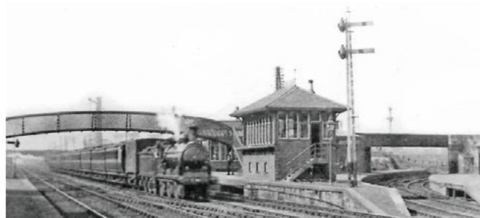
Ibrox railway station, 1849
