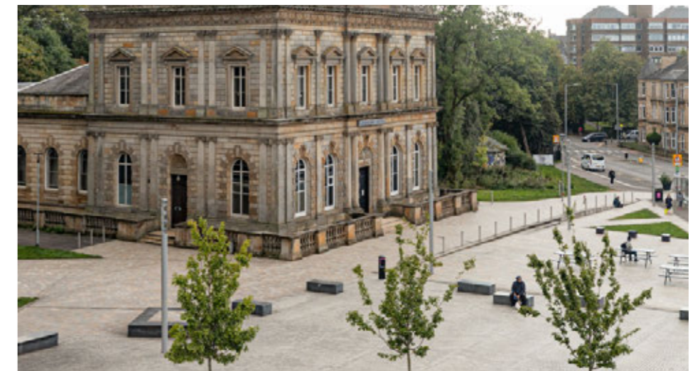
Public square with seating and planting, Shawlands Square, Glasgow
