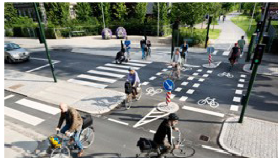
Pedestrian and cycle crossings, Green path Copenhagen
