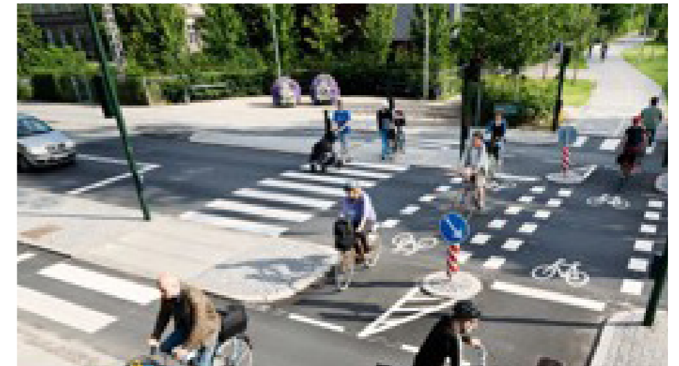
Pedestrian and cycle crossings, Green path Copenhagen
