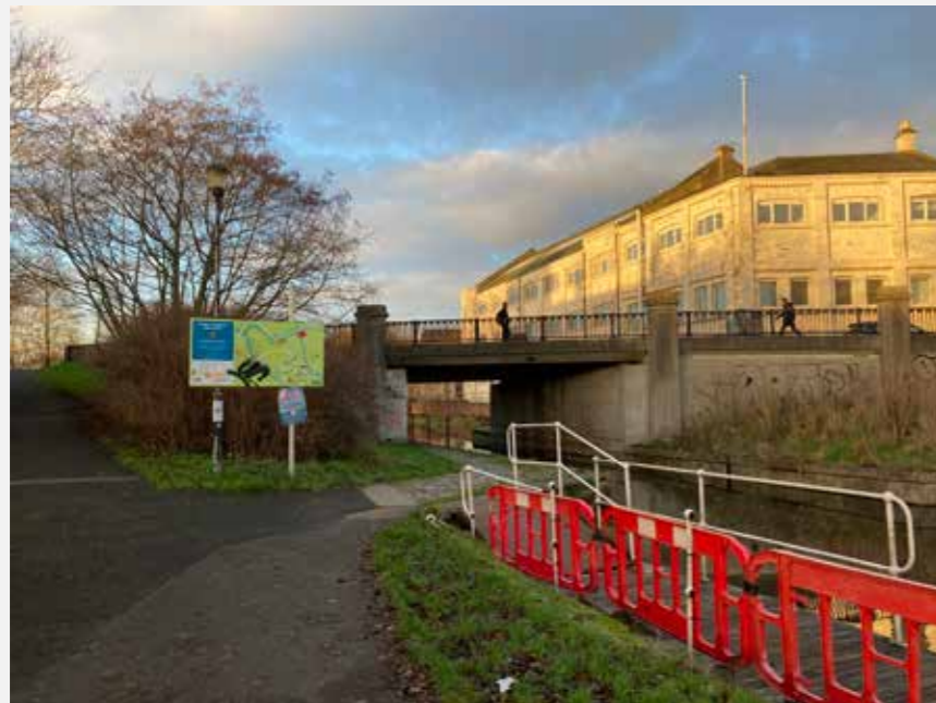
FORTH & CLYDE CANAL TOWPATH AT RUCHILL STREET ROAD BRIDGE
