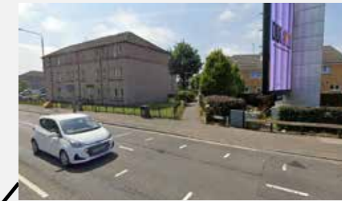
FOOTPATH ACCESS AT BALMORE ROAD
