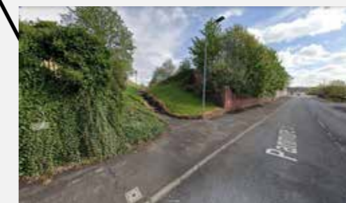
FOOTPATH ACCESS AT NORTH SIDE OF PANMURE STREET
