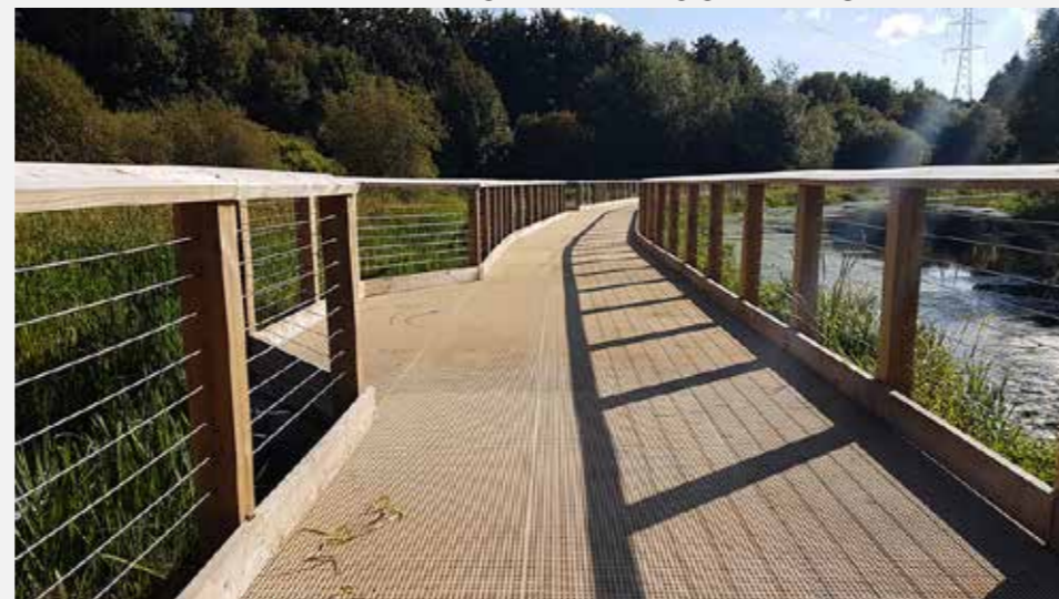
BOARDWALK FOOTWAY CLAYPITS LOCAL NATURE RESERVE
