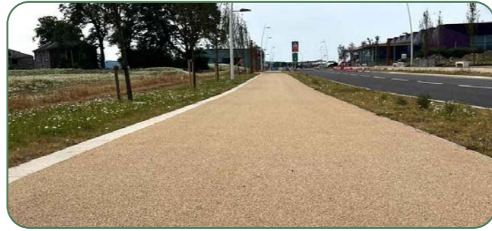
Proposed Footpaths: Neutral coloured resin bound gravel. Suitable for footpaths in green spaces and informal pathways
