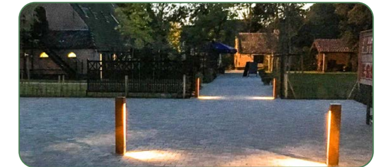
Proposed bollard lighting: Opportunities for lighting options in open spaces or along routes in the form of powder coated steel bollard lighting or similar.
