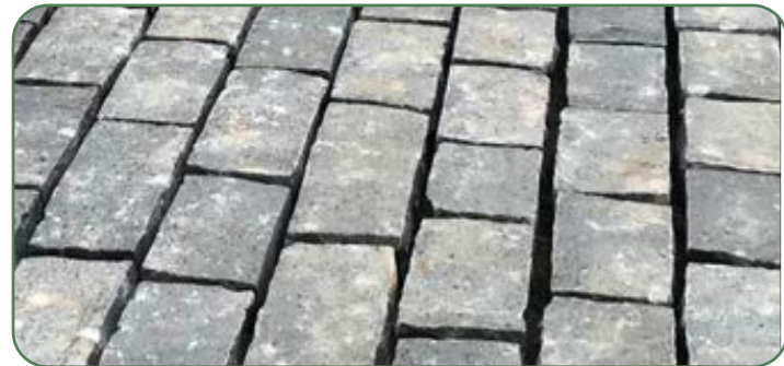
Proposed High Quality Paving: Black granite or porphyry setts as high quality natural stone option in conservation areas
