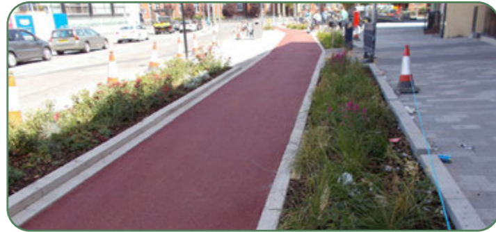
Proposed cycleways: Red coloured resin bound gravel. Alternatively red asphalt. Suitable for streetscape
