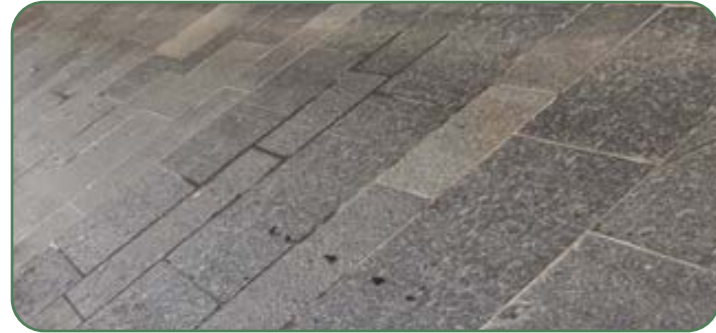
Proposed Paving: Caithness natural stone paving. Suitable for streetscape and civic spaces
