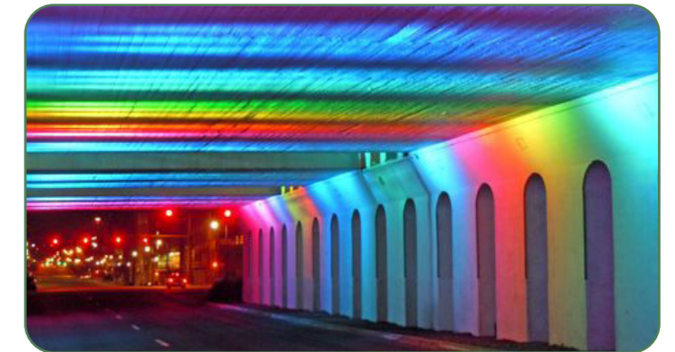
Proposed tunnel lighting: Urban light displays for safety, where active travel routes enter tunnels
