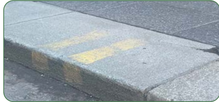
Proposed Kerbs Silver grey granite kerbs and edges. Suitable for streetscape and civic spaces
