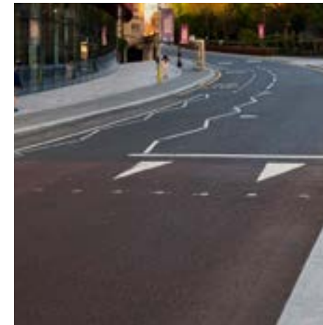
MTL-05 Asphalt with red chips Roads - raised tables
