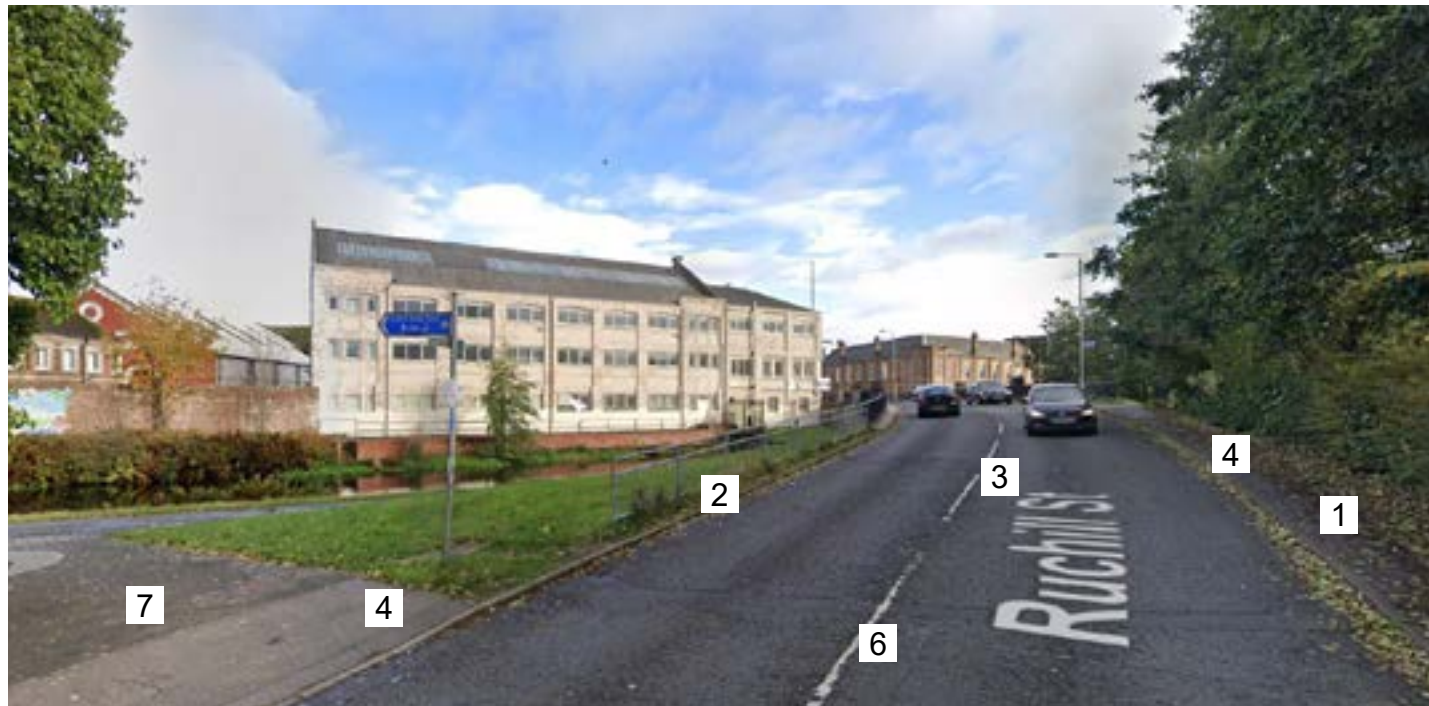
RUCHILL STREET BRIDGE APPROACH LOOKING EAST (GOOGLE)
