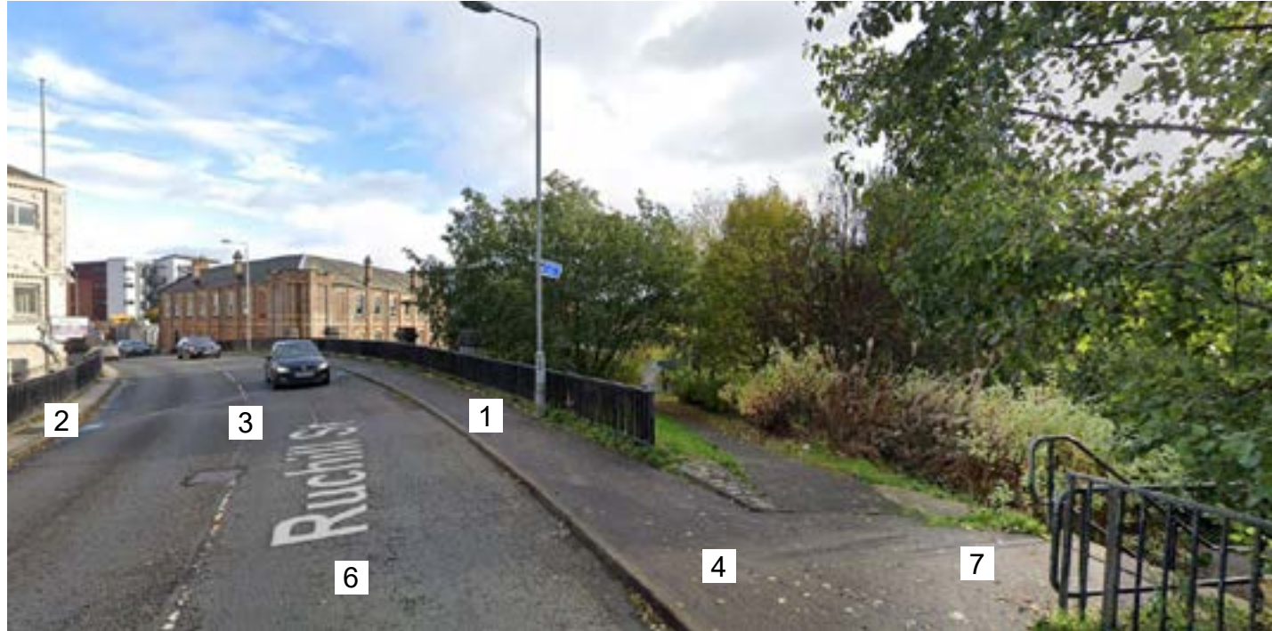
RUCHILL STREET CANAL BRIDGE (GOOGLE)
