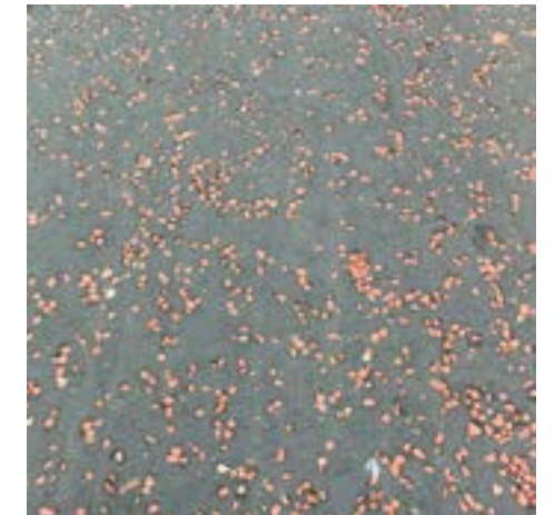
MTL-06 Asphalt with red chips Roads - raised tables
