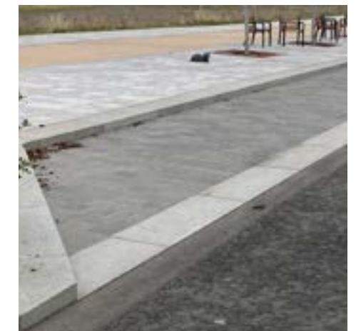
MTL-18 Block paving Parking bays
