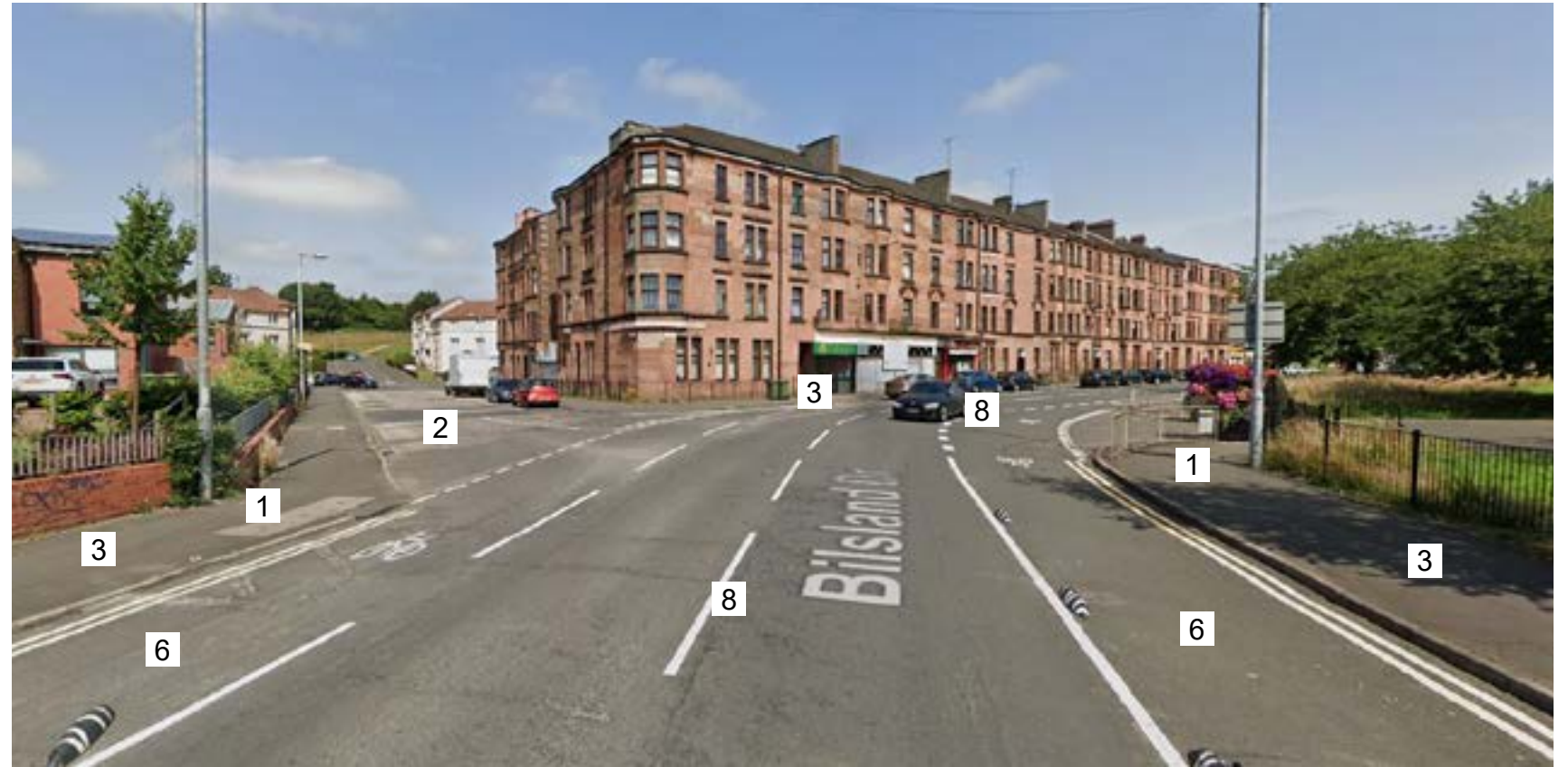
JUNCTION OF BILSLAND DRIVE & SHANNON STREET (GOOGLE)
