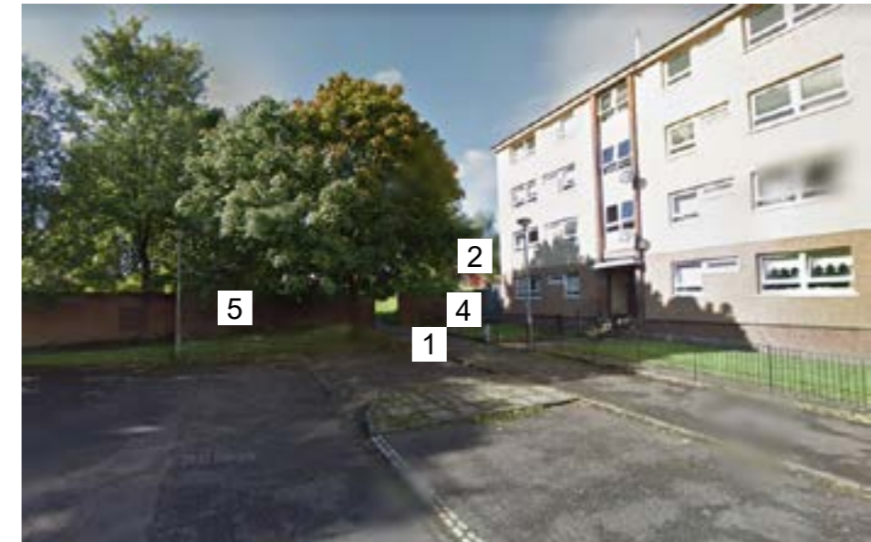
ACCESS TO DUMMY RAILWAY BILSLAND DRIVE
