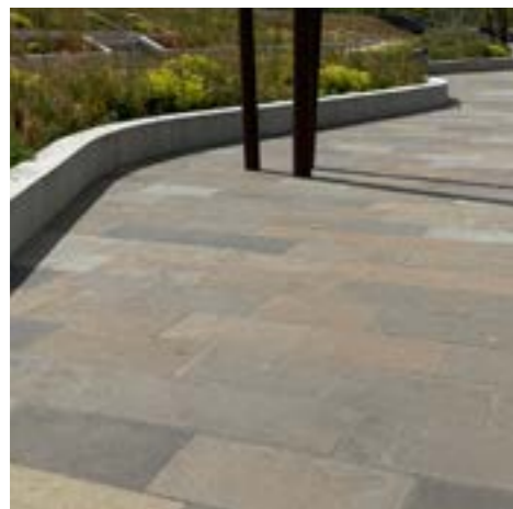
MTL-07 Natural Stone / Caithness Pedestrian crossings
