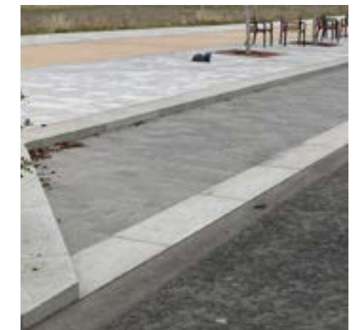
MTL-18 Block paving Parking bays
