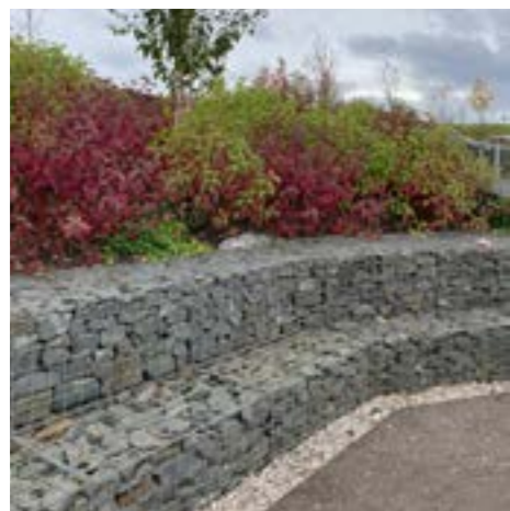
Gabion landscaping Sighthill, Glasgow
