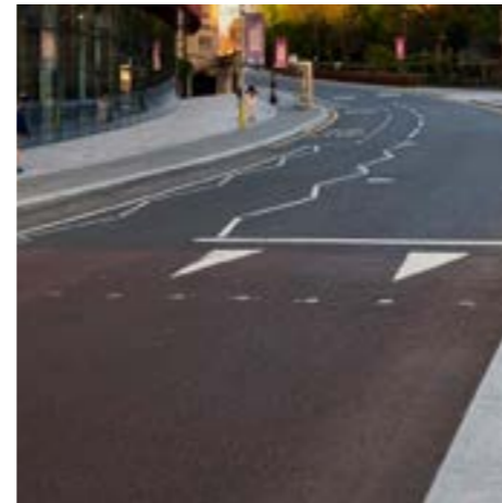
MTL-03 Asphalt with red chips Roads - raised tables
