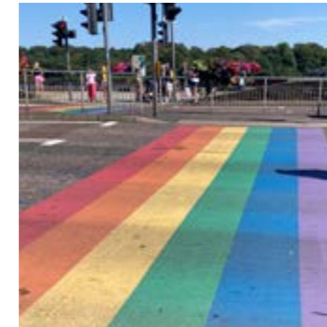
MTL-05 Asphalt with Cold Plastic Road Marking paint Crossing point on raised table
