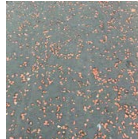
MTL-04 Asphalt with red chips Roads - raised tables
