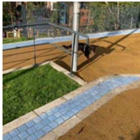
MTL-09 New Path through green space – Allow for Resin bound gravel / porous surface
