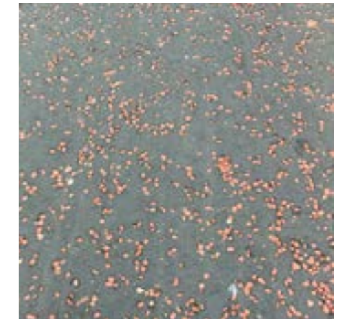
MTL-06 Asphalt with red chips Roads - raised tables
