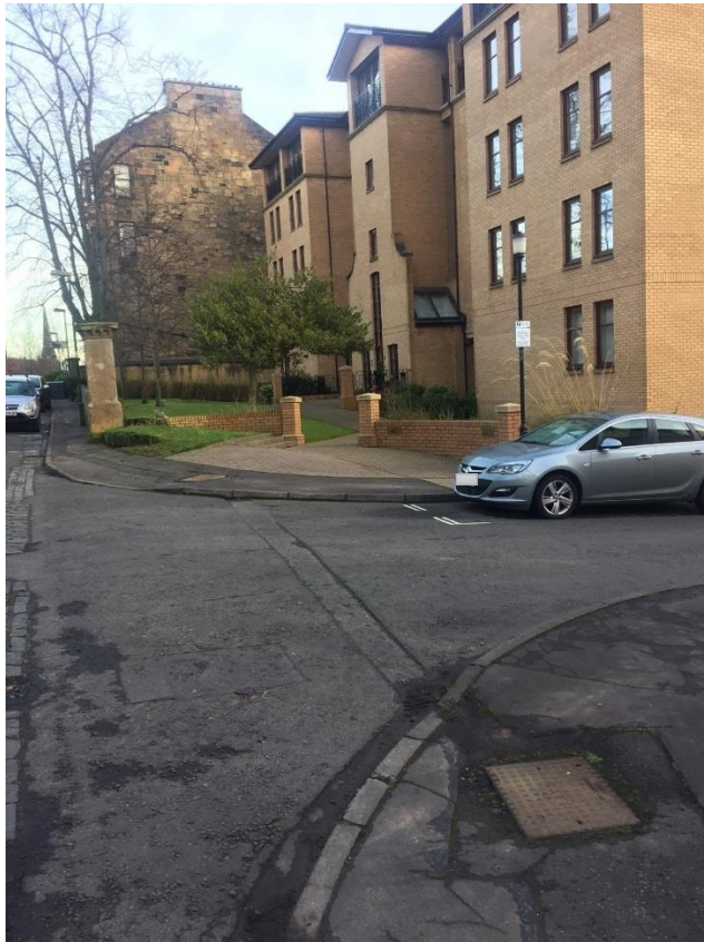
Partickhill Road Access Road (after)
