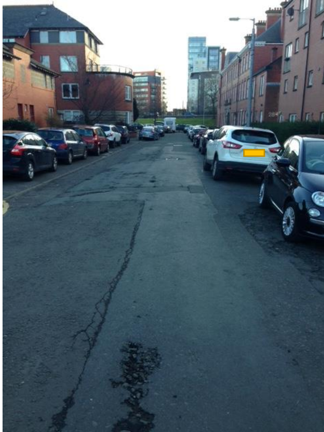
Sandy Road (before)
