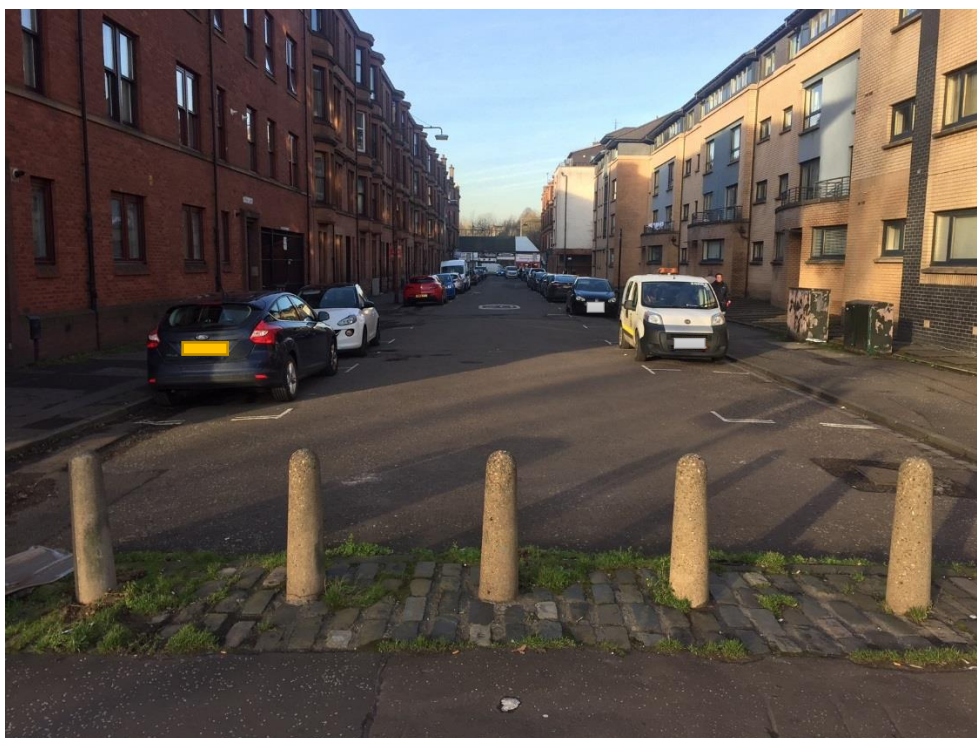
Hayburn Street (after)
