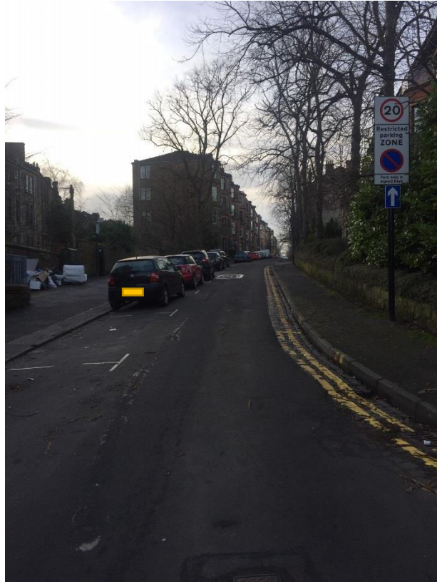
Partickhill Road (after)
