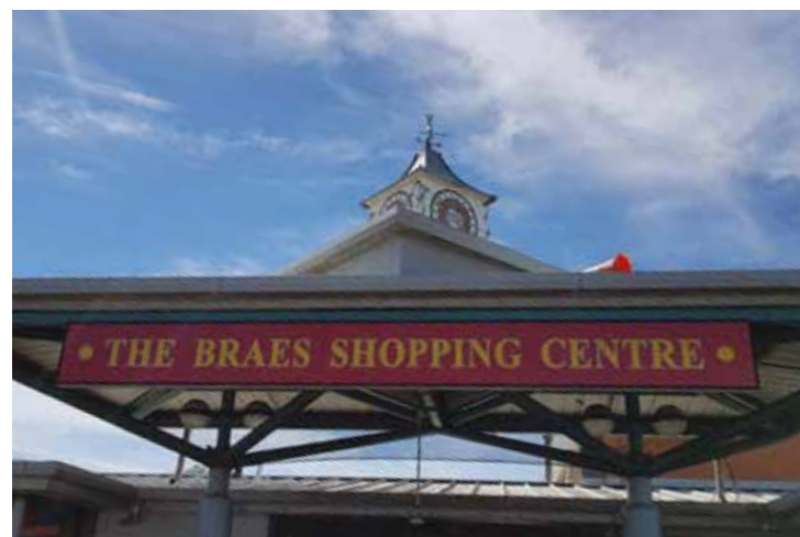
Figure 8: The Braes Shopping Centre, retail attractor
