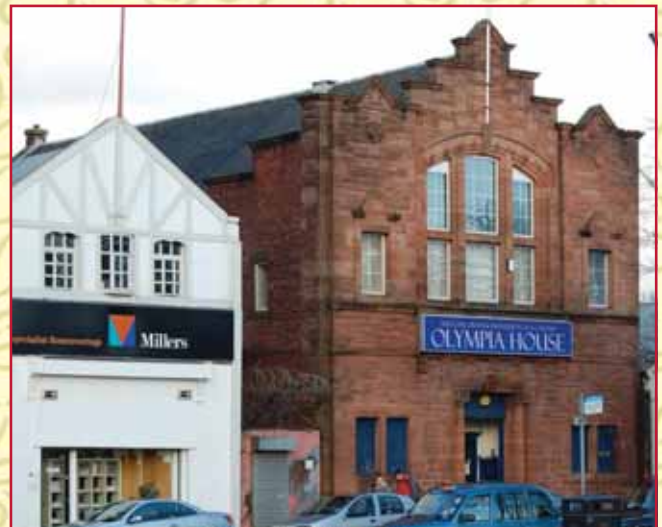
Former Salvation Army Hall, Olympia Street
