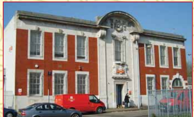
Telephone Exchange, Cubie Street
