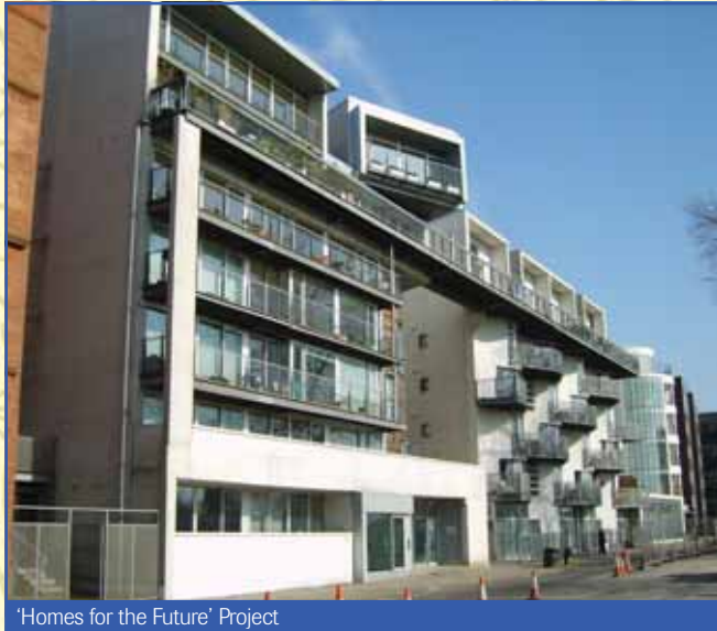
'Homes for the Future' Project
