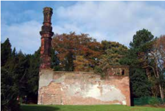
Chimney stalk and remains of boiler house
