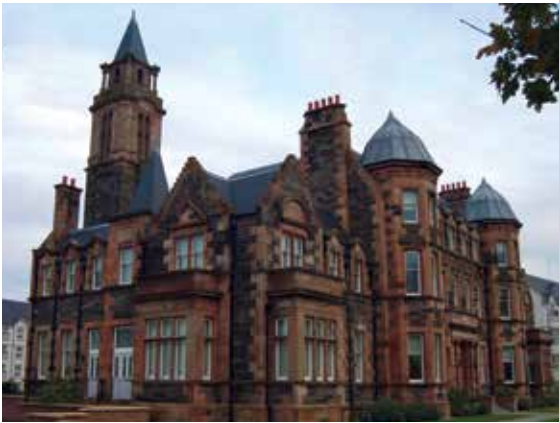
Leverndale Hospital Towerview Unit with water tower behind
