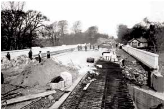
New Howford Bridge under construction 1933 with Ross Hall South Lodge
