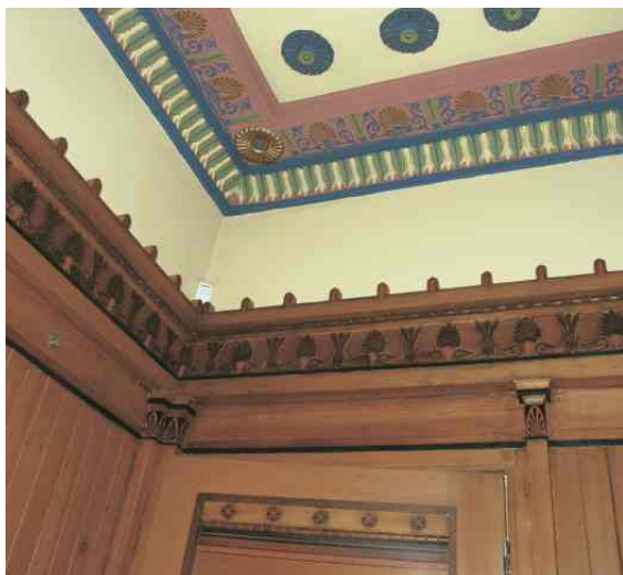
Interior detail, Double Villa
