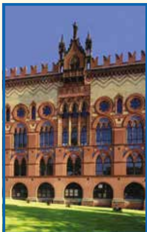
Exquisite Brickwork on Main Façade of Templeton's Carpet Factory
