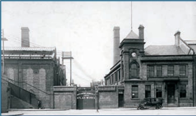
Atlas works Springburn
