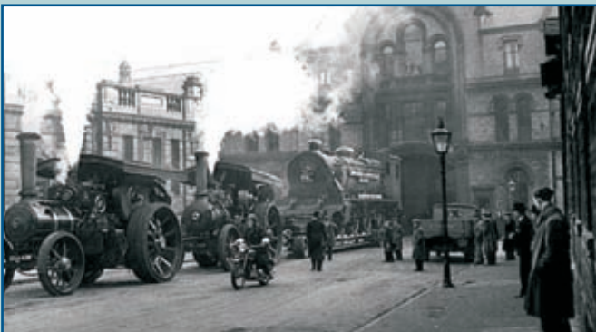
Locomotive leaving Hyde Park works
