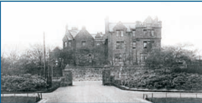
The Reid home Belmont House
