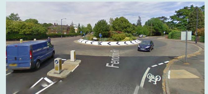
Figure 4.62: Before image of a roundabout in Cambridge.
