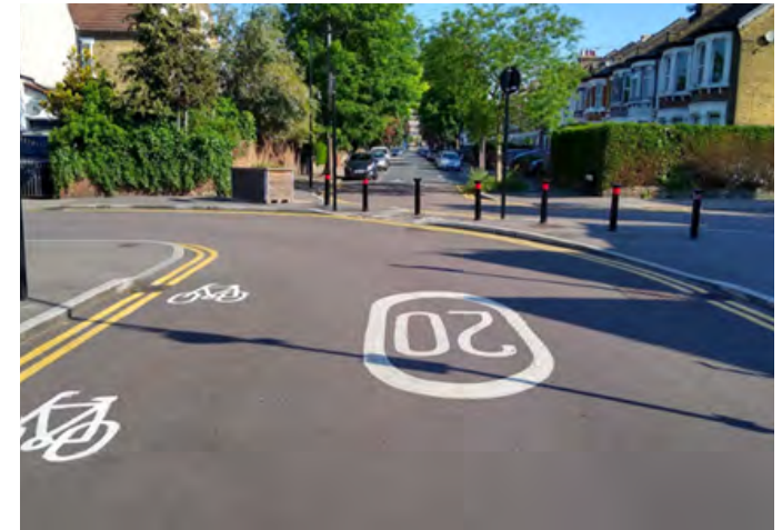
Figure 4.27: Ground view of the new modal filter from figure 4.26.
