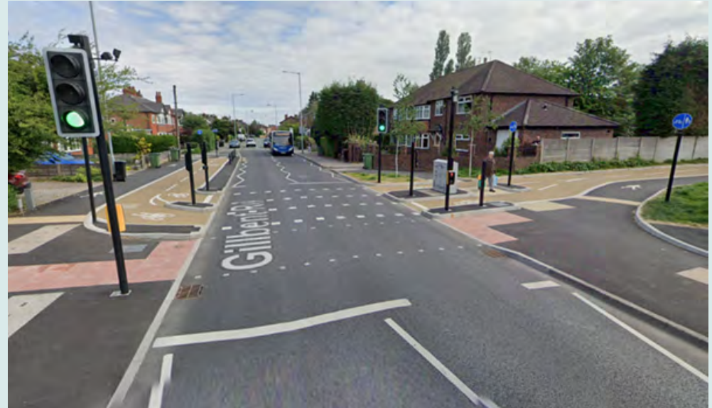
Figure 4.50: after image of crossing which has protected cycleway crossing alongside pedestrian crossing.
