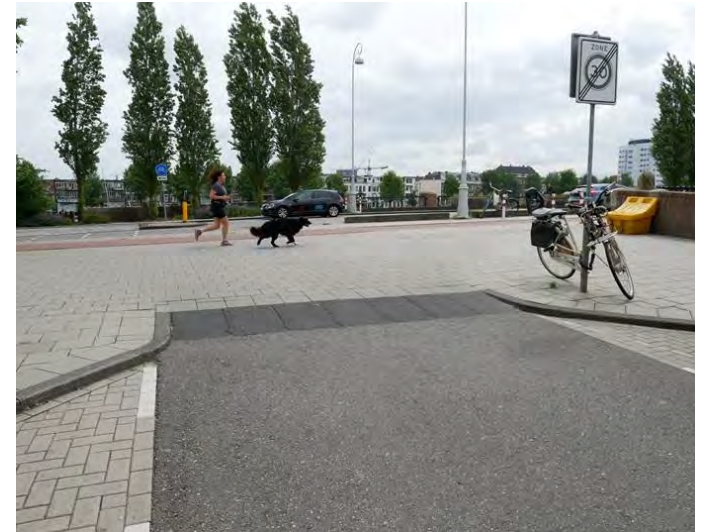
Figure 4.45: Example from Netherlands of continuous footway across side street junction. A person is running with their dog across the footway.
