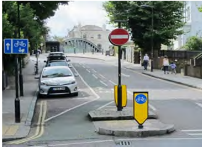
Figure 4.30: Contraflow cycle lane with island separator to better protect people cycling at the junctions.
