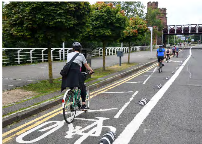
Figure 4.9: People using protected cycle space introduced on Clyde Street as part of Spaces for People.
