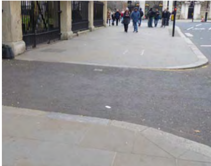
Figure 4.43: Example from Glasgow of side street junction where road is raised to footway level.
