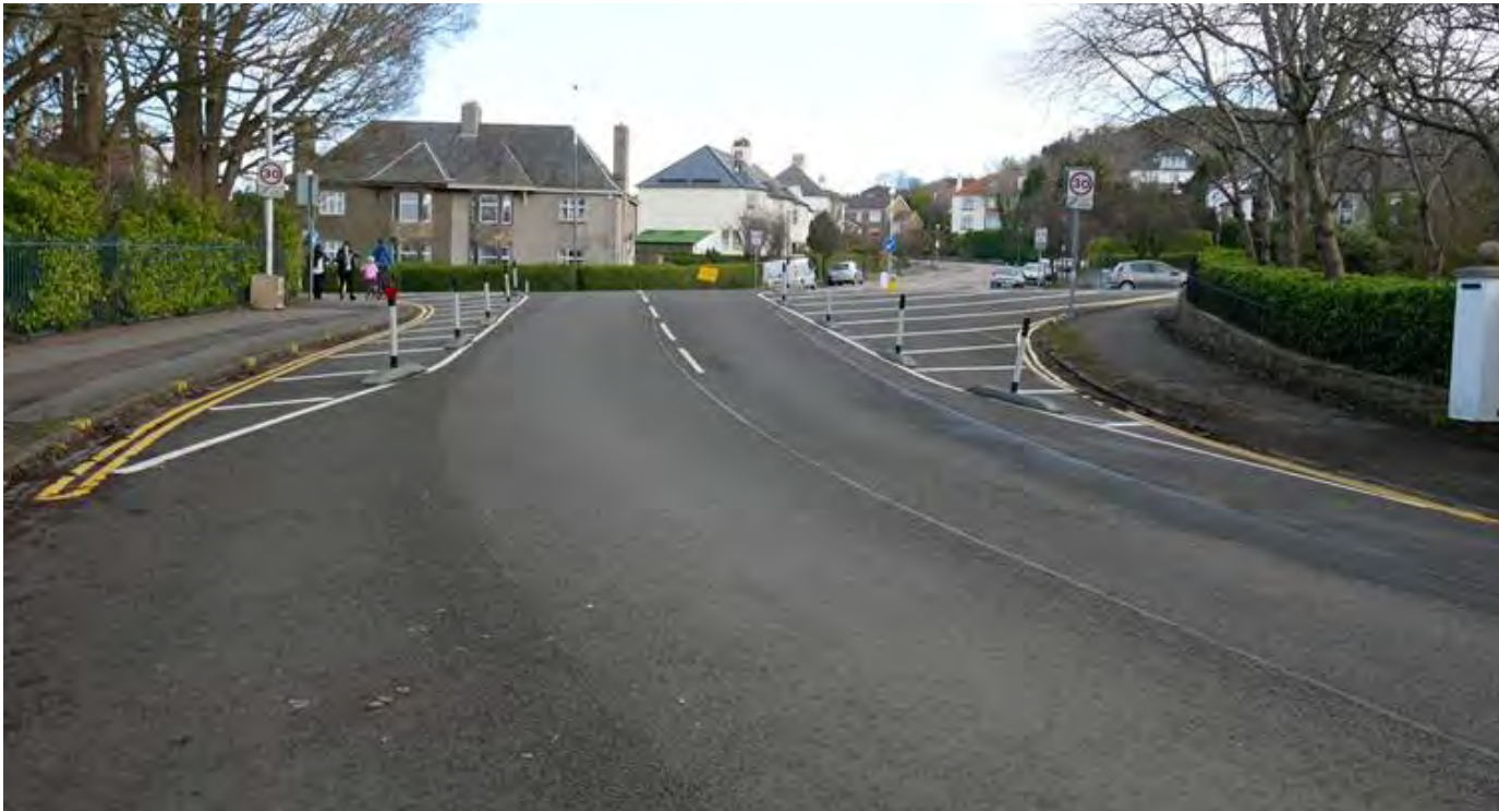
Figure 4.41: Side street junction in Edinburgh where paint and bolt down bollards have been used to significantly reduce road width to create safer pedestrian crossing environment.
