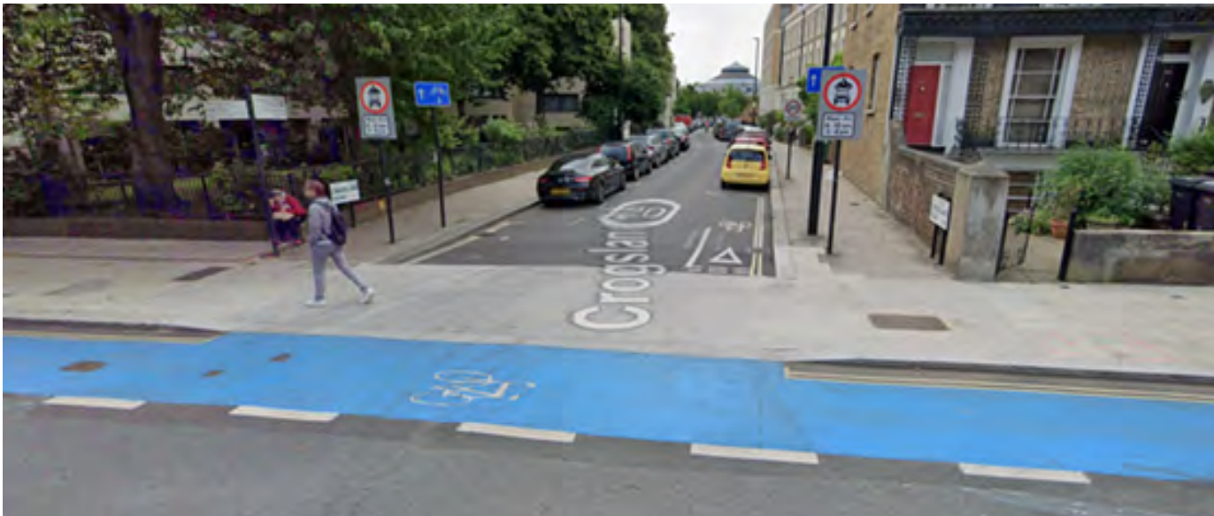
Figure 4.42: Example of continuous footway across a side street junction in London with someone crossing. Foreground shows blue coloured cycleway.
