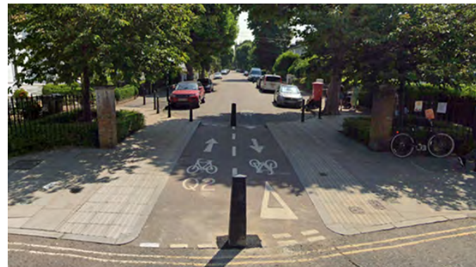
Figure 4.21: Example of side street modal filter in London which has designated cycleway.
