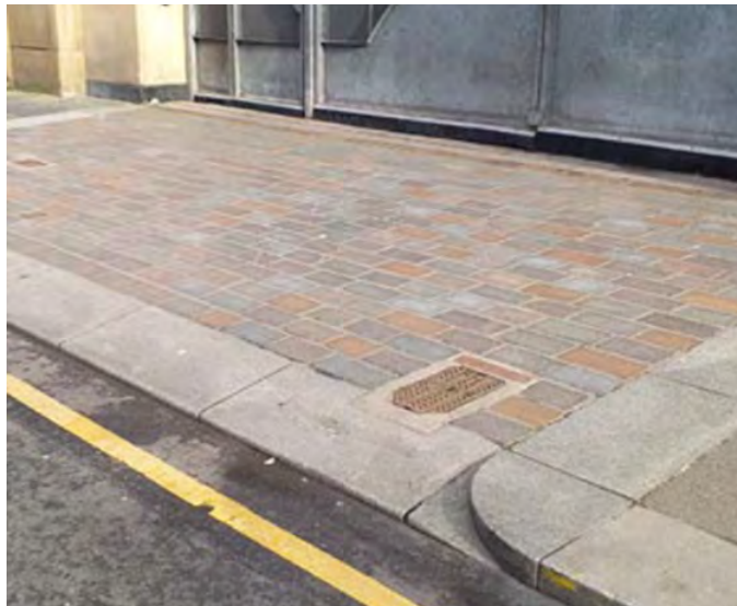
Figure 4.44: example from Glasgow of Side Street junction where high quality paving is used with steep ramp up to slow vehicles.
