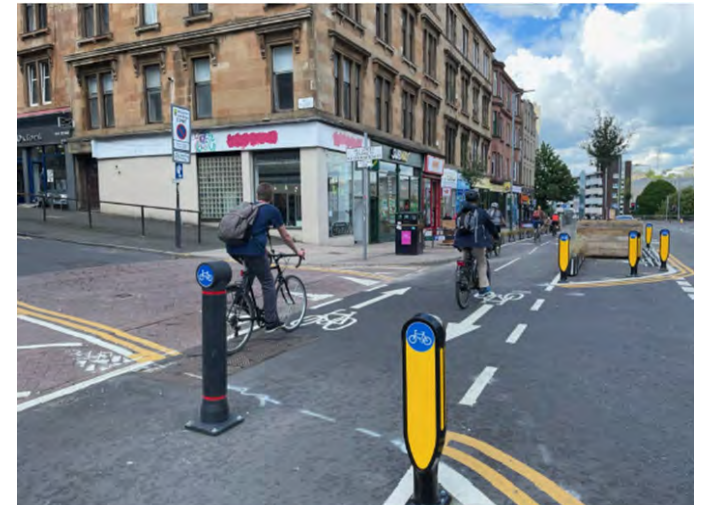
Figure 2.16: Cambridge Street with people cycling across a side street using the cycleway. Bollards were added to Cambridge Street alongside bolt down cycle infrastructure.
