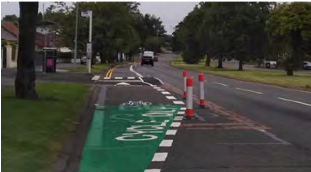
Figure 4.15: Great Western Road with space for people cycleway showing bus stop build out.
