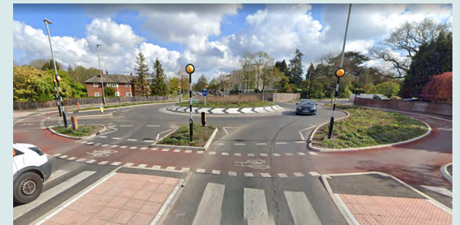
Figure 4.63: After image of cycleway and pedestrian zebra crossings added to roundabout.
