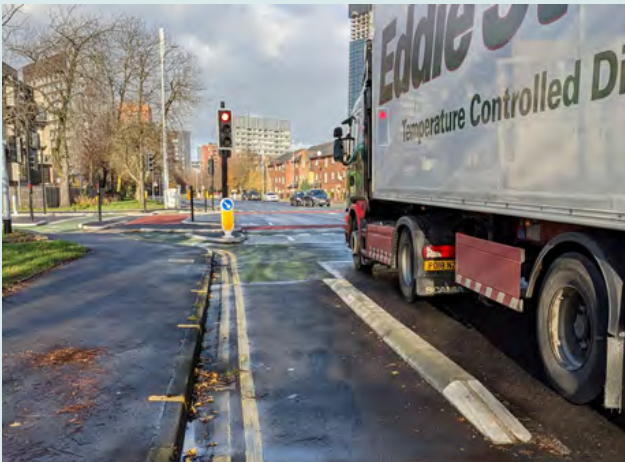
Figure 4.55: Bolt down kerbs leading to protected cycling junction in Manchester. Large HGV is waiting at lights but junction layout means those cycling do not have to interact with motor traffic.
