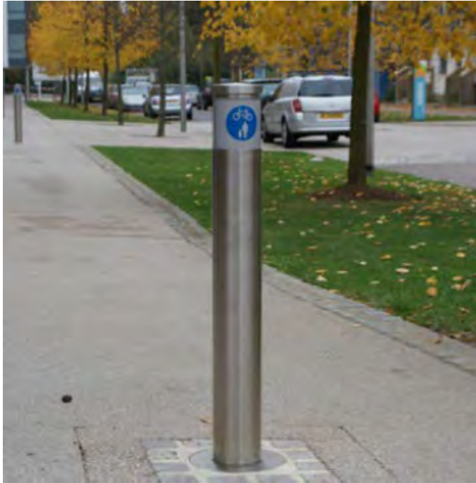
Figure 4.83: Bollard with small blue sign to denote shared use path.
