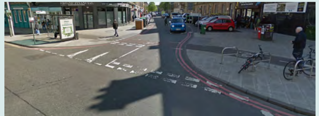
Figure 4.35: Side street junction in Edinburgh where road marking and a raised table are used to give people cycling and walking priority.
