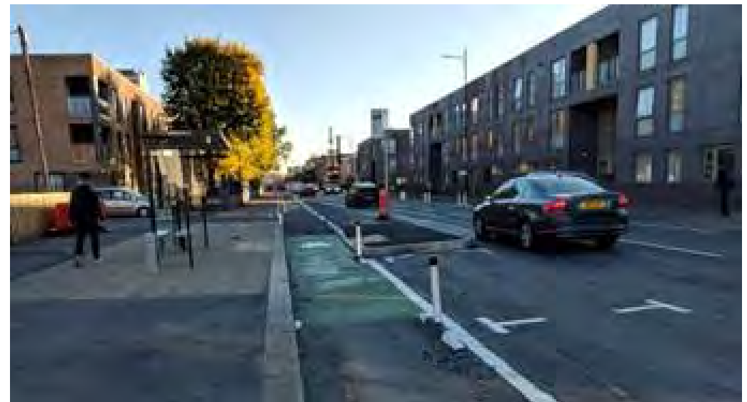
Figure 4.16: Bus stop island in Manchester with separated people boarding and alighting the bus from those cycling.
