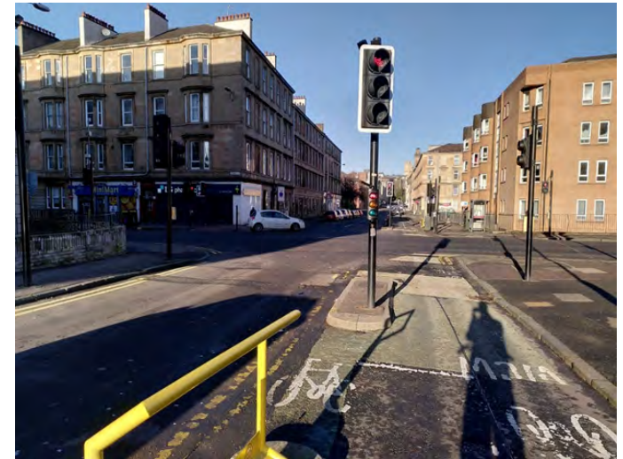
Figure 2.9 Protected cycleway with signalled junction with dedicated cycle phase on West City Way.
