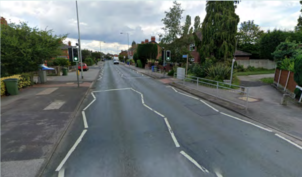
Figure 4.49: before image of standard pedestrian crossing.
