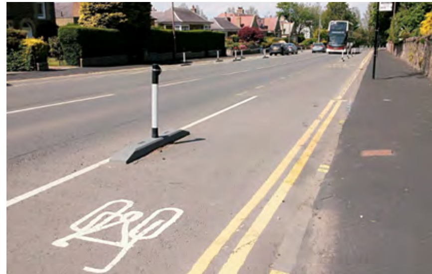
Figure 4.14: Spaces for People cycle provision in Edinburgh with bolt down bollards to protect the cycleway.
