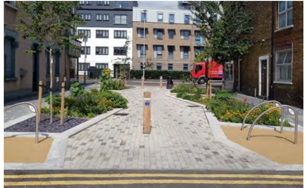
Figure 4.24: After image of side street junction after new light colour paving greenery and cycle hoops have been added.
