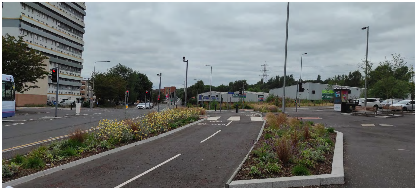
Figure 3.1: Remodelled junction on Garscube Road, road space has been reallocated to introduce greenery, a cycleway, and extended pedestrian plaza with benches.
