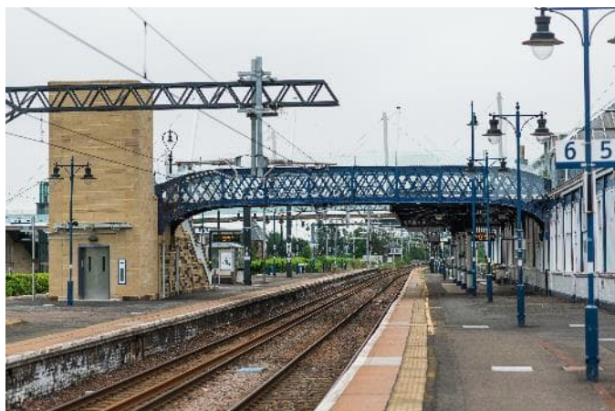
Source: Network Rail
