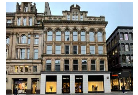
71-79 Buchanan Street 3 Upper storeys over retail
