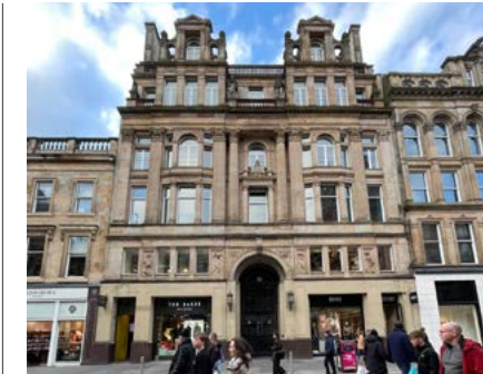
61-79 Buchanan Street 3 Upper storeys over retail
