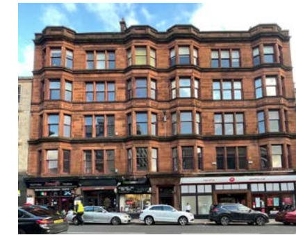
136-146 West Nile Street 4 Upper storeys over retail
