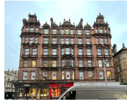
116-128 Buchanan Street 5 Upper storeys over retail
