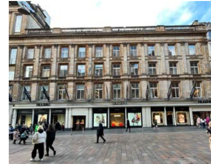
21-45 Buchanan Street 4 Upper storeys over retail
