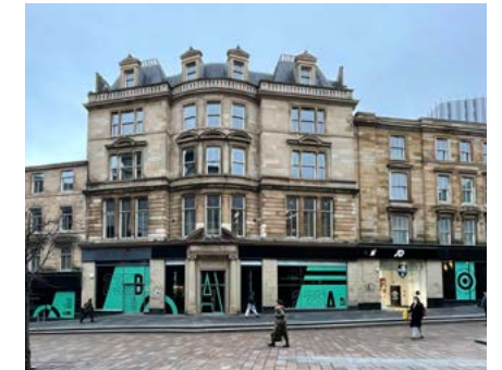
235-249 Buchanan Street 3 Upper storeys over retail
