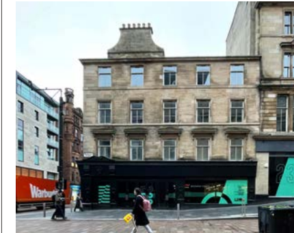
229 Buchanan Street 2 Upper storeys over retail
