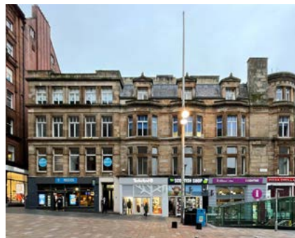
156-164 Buchanan Street 3 Upper storeys over retail
