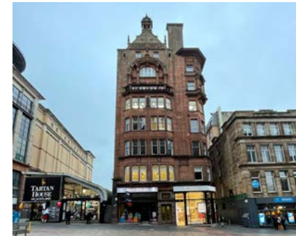
164-168 Buchanan Street 6 Upper storeys over retail
