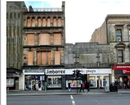
137-149 Trongate 1-3 Upper storeys over retail
