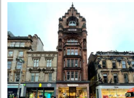
60-62 Buchanan Street 2-5 Upper storeys over retail
