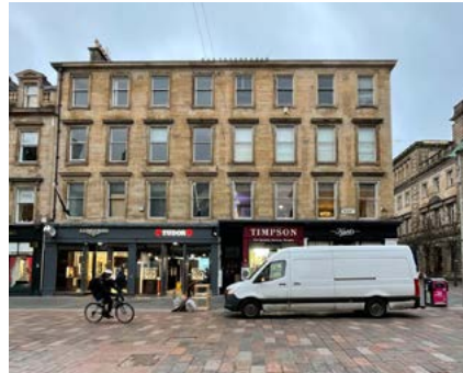
101-111 Buchanan Street 3 Upper storeys over retail
