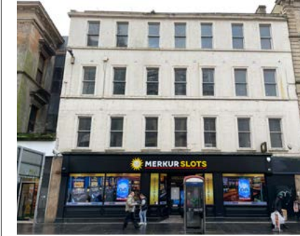
159-163 Trongate 3 Upper storeys over retail
