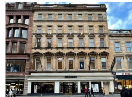
55-59 Buchanan Street 4 Upper storeys over retail
