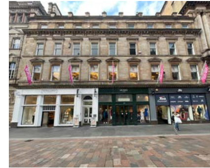
123-129 Buchanan Street 3 Upper storeys over retail
