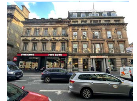
57-65 St. Vincent Street 3 Upper storeys over retail
