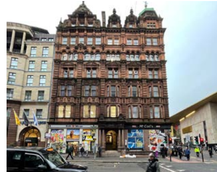
34-38 West George Street 2 Upper storeys over retail
