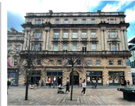
131-137 Buchanan Street 3 Upper storeys over retail
