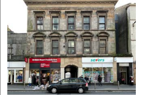
151-157 Trongate 2 Upper storeys over retail
