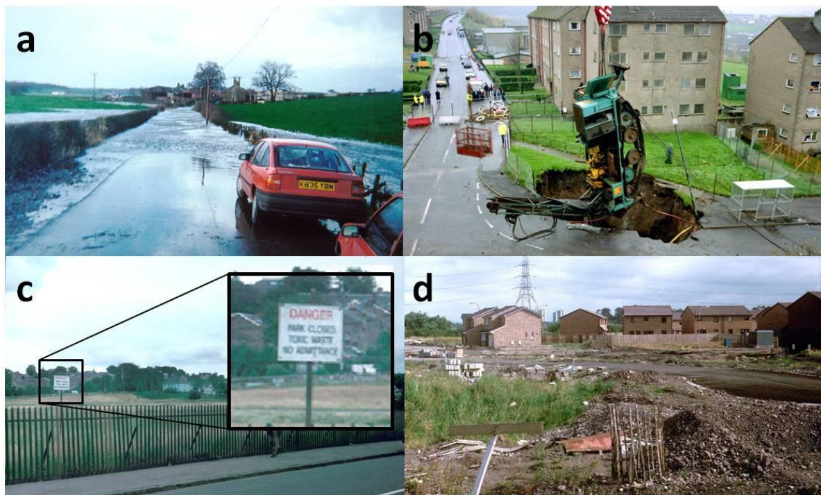
Figure 4 Photographs from Glasgow showing (a) groundwater flooding, (b) catastrophic collapse of a mine shaft resulting in loss of a drilling rig, (c and d) contaminated and derelict ground.
