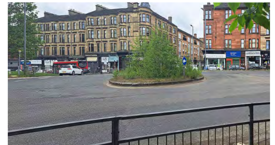
Existing: Dumbarton Road / Victoria Park Drive South roundabout
