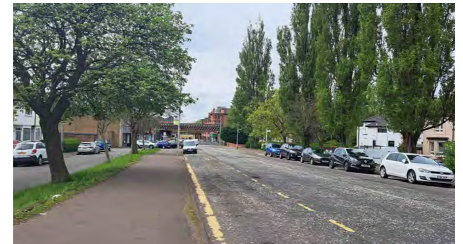
Existing: Anniesland Road, looking towards Dumbarton Road
