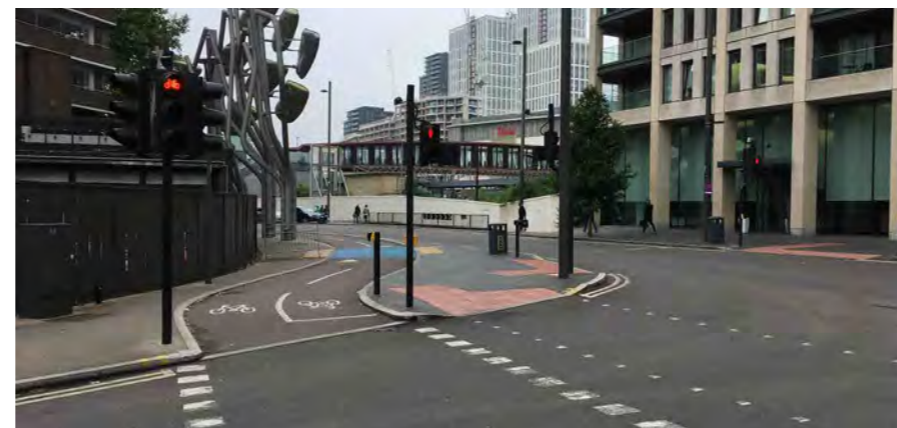
Precedent: Segregated cycle lanes at a junction in Stratford, London
