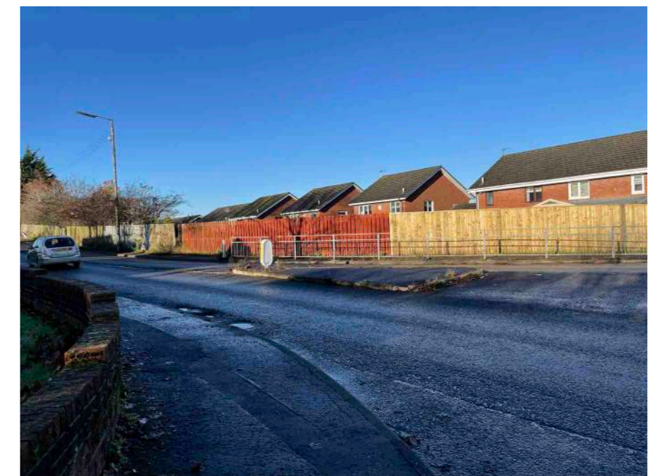
Lack of crossing facility at a roundabout on Royston Road (Hogganfield) and guardrailing blocks crossing on the desire line.
