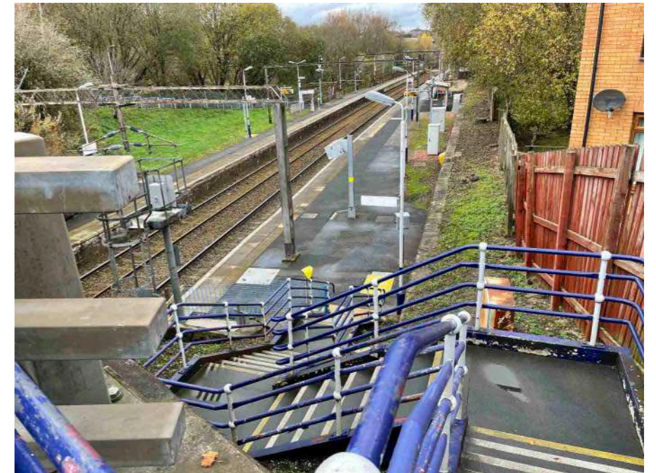
Barnhill Station lacks step-free access.
