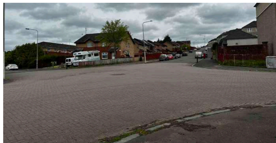
Forge Street - existing
