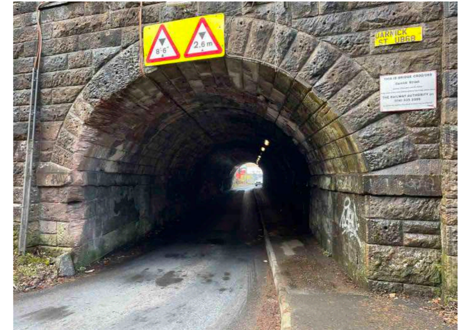
Blind Tunnel at Darnick Street
