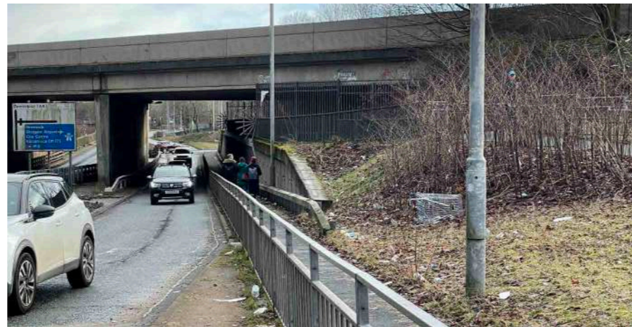
Route alongside Viewpark Avenue - existing
