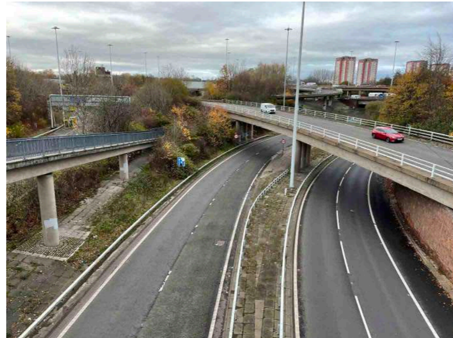
Junction 15 of the M8 motorway is a key severance feature, hindering access to the city centre.
