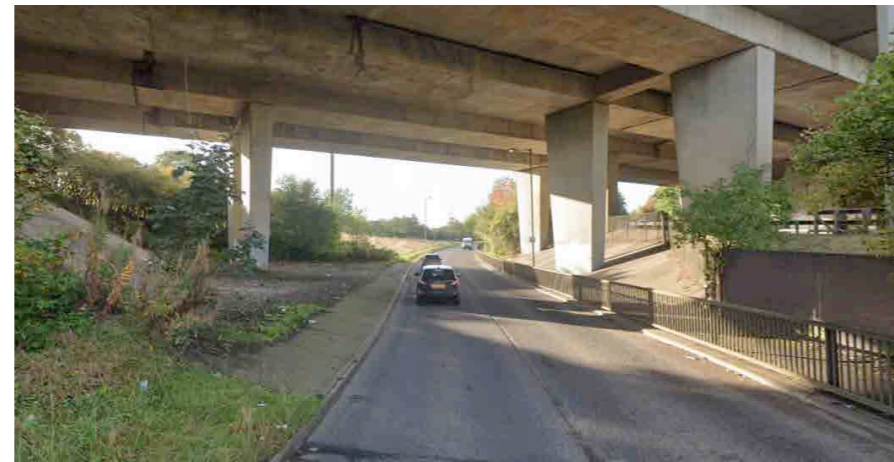
Junction 13 slip road
