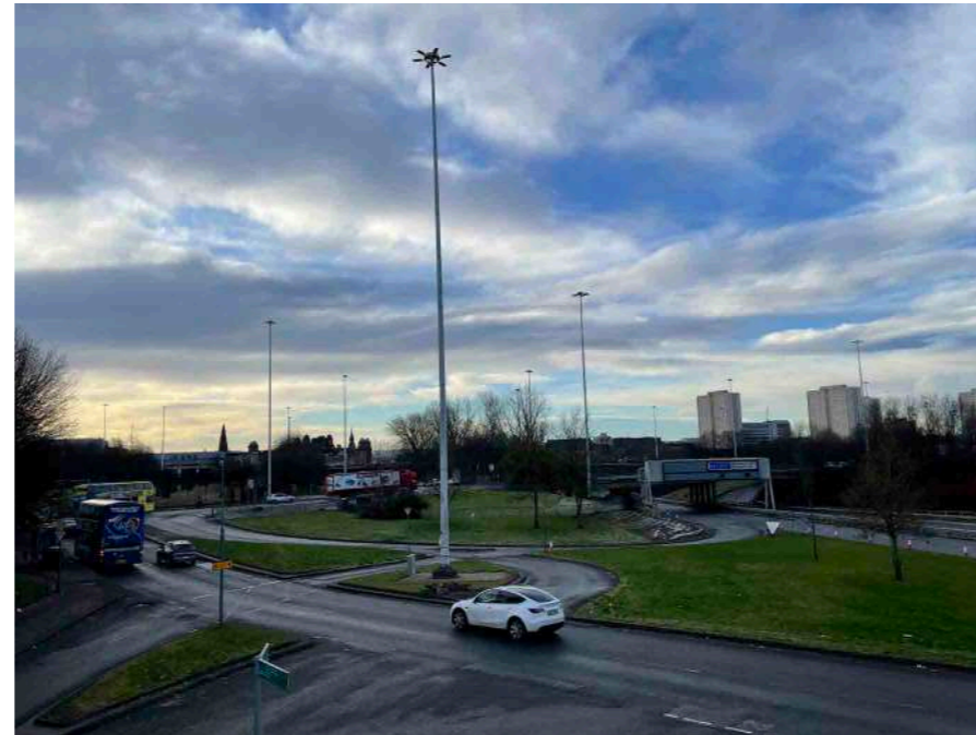
Junction 15 occupies a vast amount of land, and results in many leftover verge spaces.
