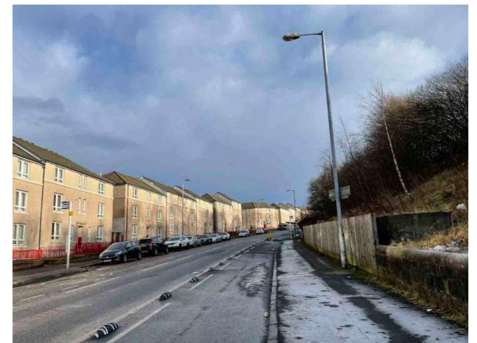
Royston Road (Germiston) provides a bi-directional light segregated cycle track.
