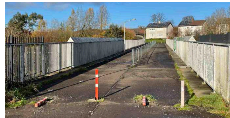
Existing bridge to Winifred
