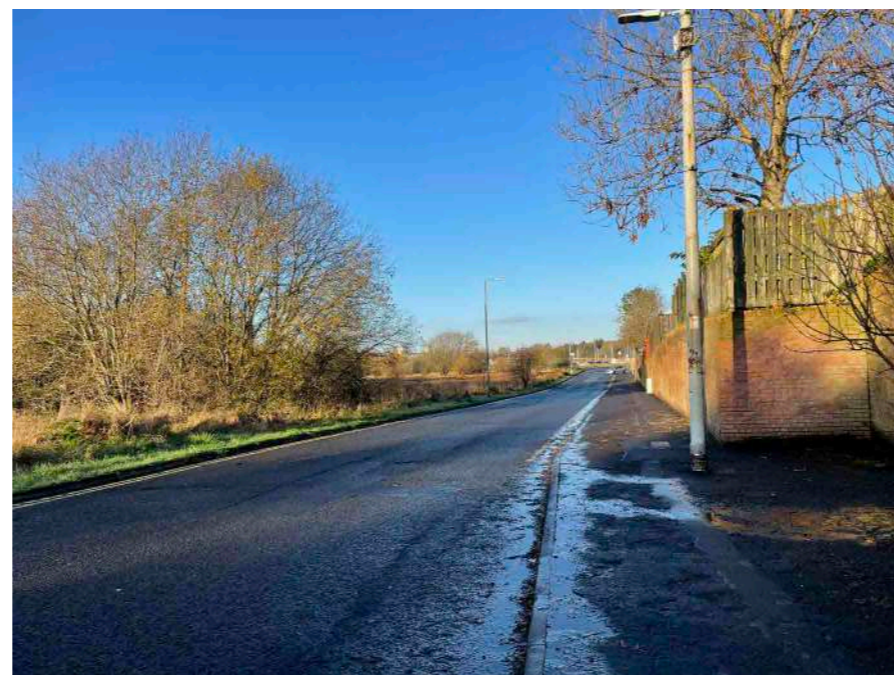
Station Road (Hogganfield) provides a link between Hogganfield and Robroyston Station.
