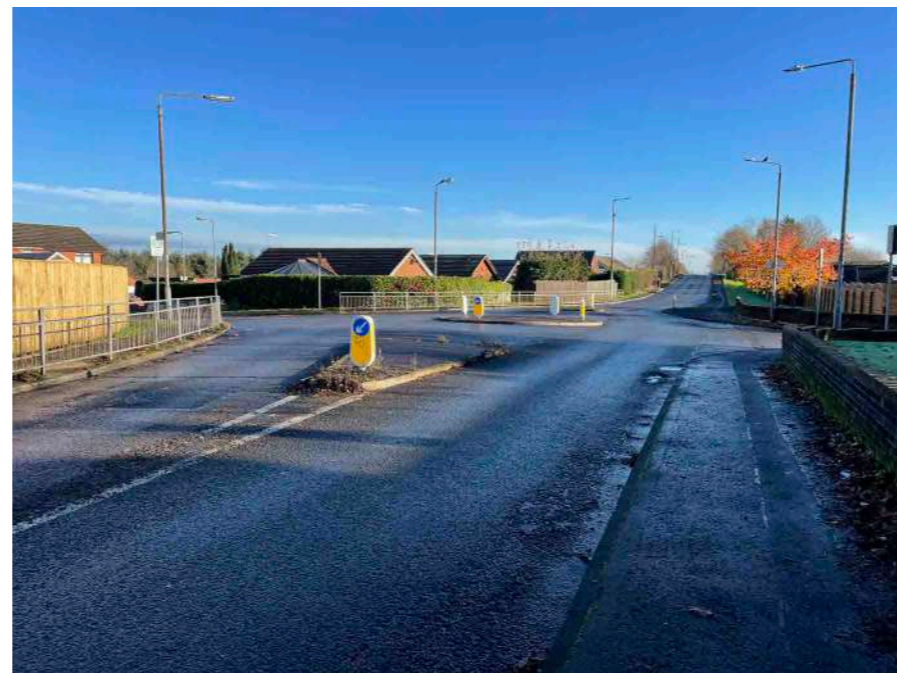
This roundabout on Royston Road (Hogganfield) lacks any pedestrian crossing provision, and prevents informal crossing on the desire line with guardrailling.
