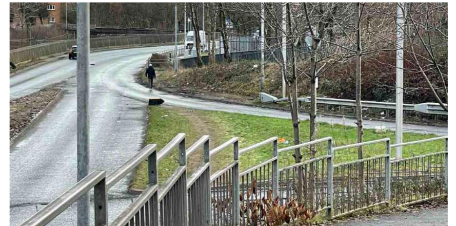
Desire line crossing of M8 sliproad - Viewpark Avenue - existing
