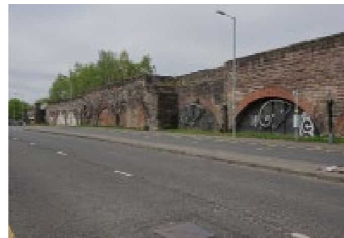
Figure 46: Blocked up railway arches
