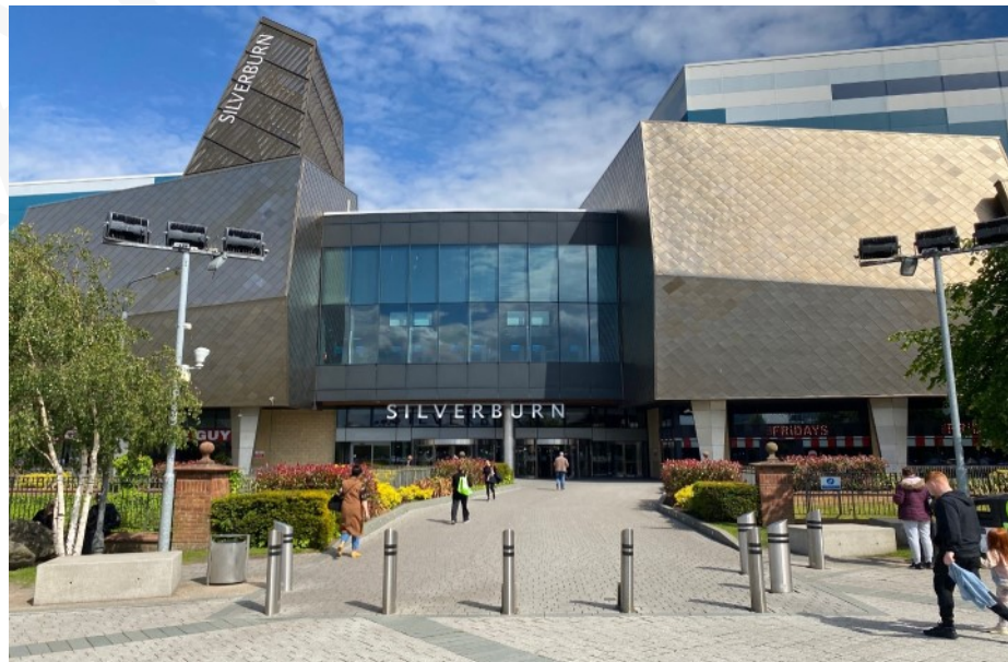
Silverburn Shopping Centre West Entrance
