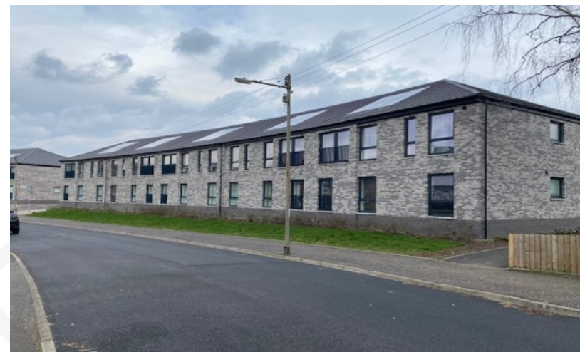
Damshot Road new homes: Old Pollok
