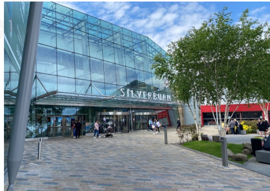
Image of Silverburn Shopping Centre via Eastern Entrance
