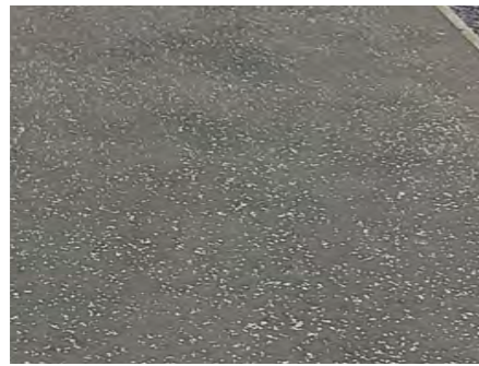
Proposed footway (standard asphalt): Bituminous Macadam
