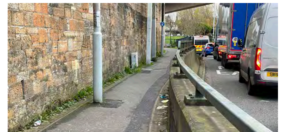
Narrow pinch point on Springburn Road shared use footway.
