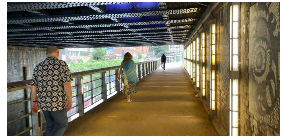
Underpass lighting integrated into the supporting wall.
