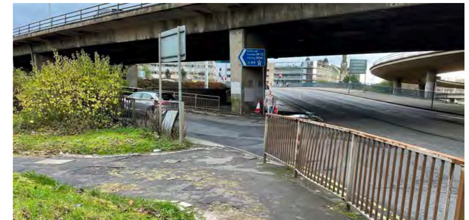
Lack of crossing points at the M8 slip road junctions.
