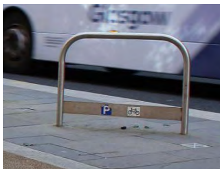
Cycle stands: Silver galvanised steel clip Sheffield stands (Cycling by Design 2021) 2
