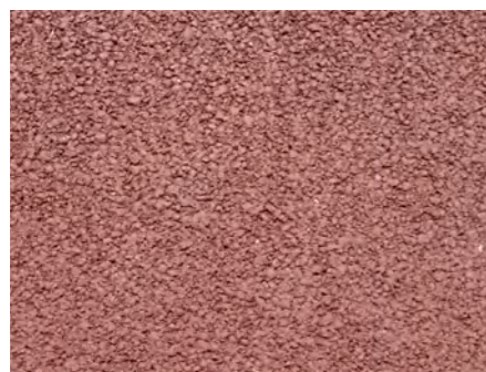
Carriageway narrowing: Red asphalt
