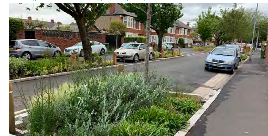
Raised table side road junction.
