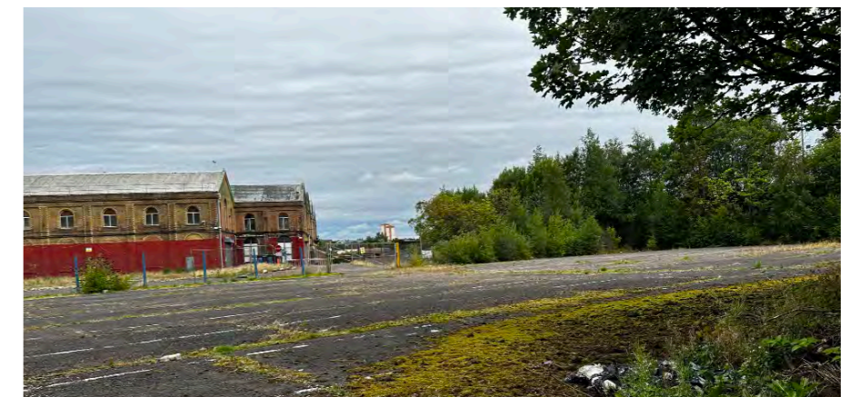
Former railway works.
