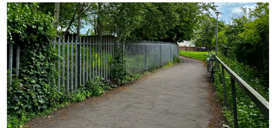
Lack of access to St Joseph's Court due to existing fencing.
