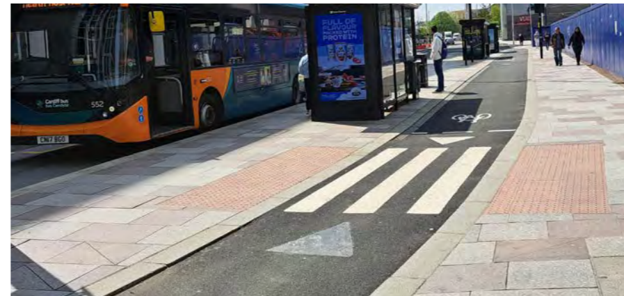
Precedent: tactile paving at a pedestrian crossing
