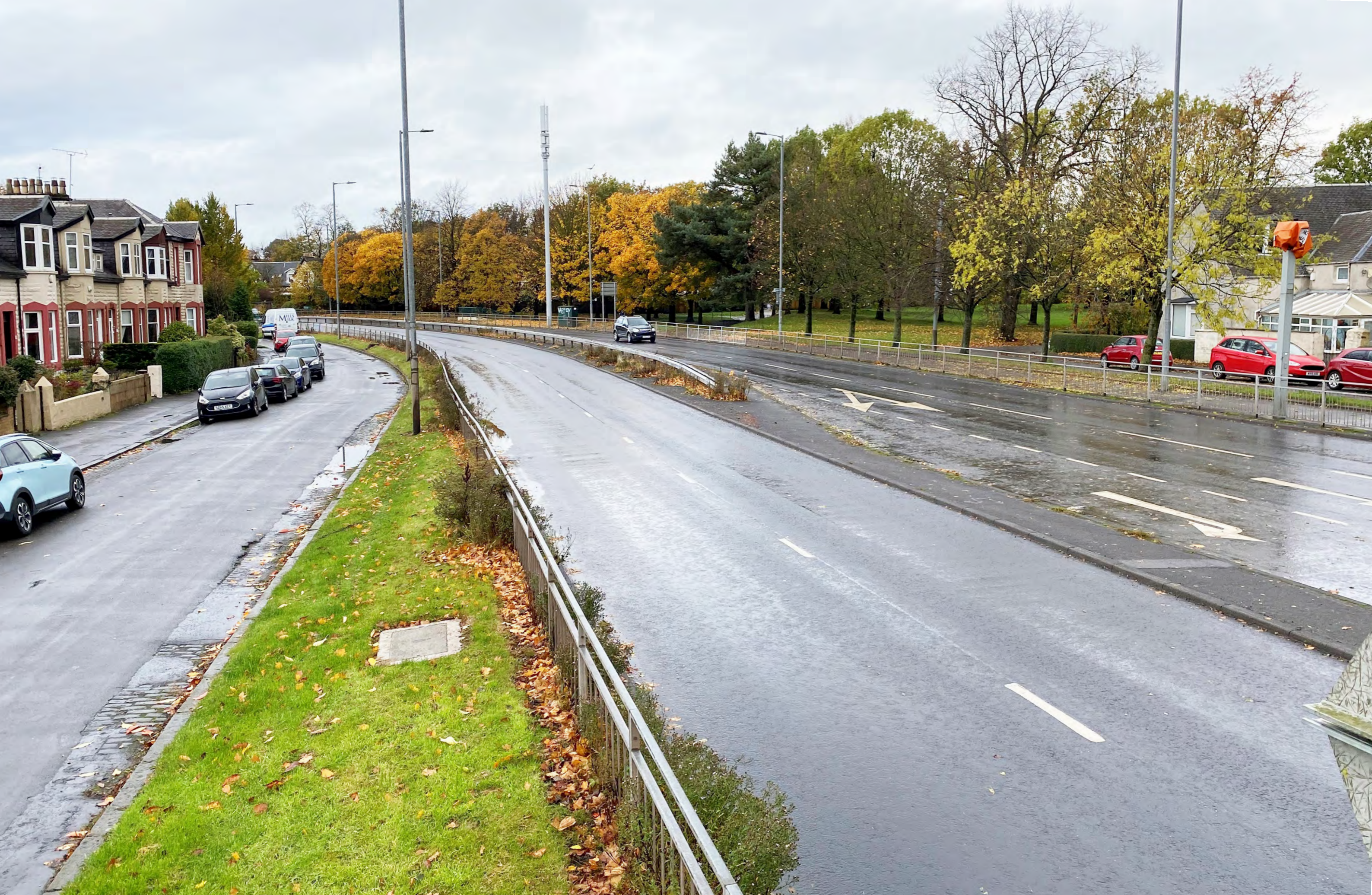
View of the current situation at Victoria Park Drive South (West)
