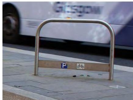
Cycle stands: Silver galvanised steel clip Sheffield stands (Cycling by Design 2021) 2
