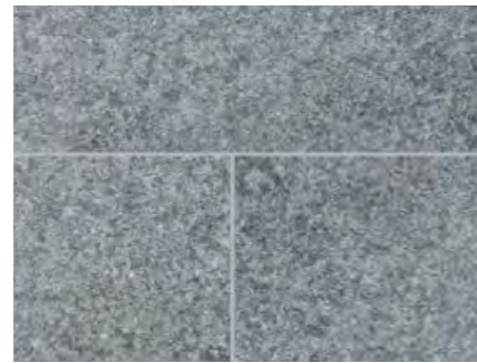
Continuous footway: Mid/Dark Grey Smooth Ground Concrete Flag. Paving with Natural Stone Aggregate 1
