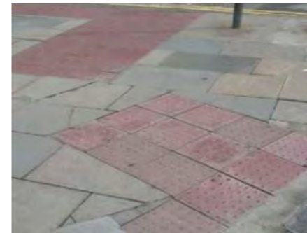
Tactile paving (blister): Blister concrete paving slabs - 400x400 in red 1
