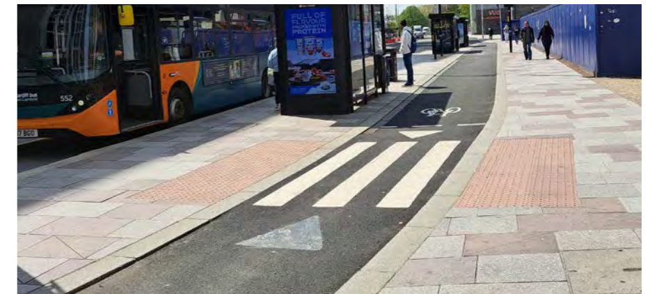
Precedent: tactile paving at a pedestrian crossing
