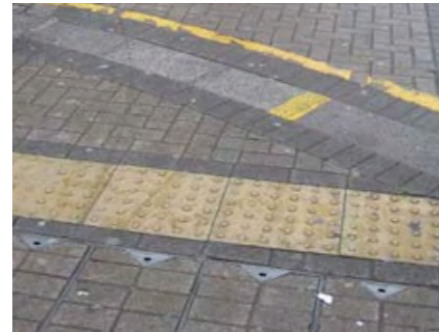
Tactile paving (blister): Blister concrete paving slabs - 400x400 in buff 1
