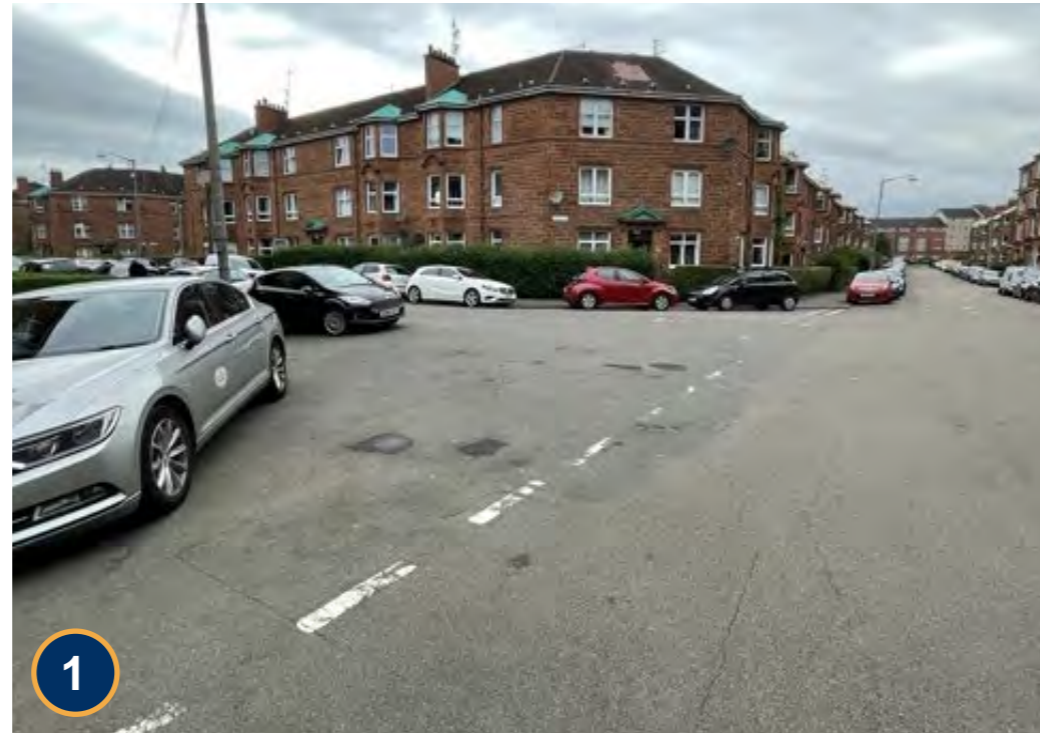
1 Extremely wide bell-mouths which encourage obstructive parking behaviours
