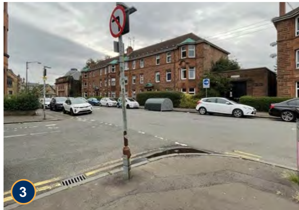
3 Poor visibility and drainage issues.
