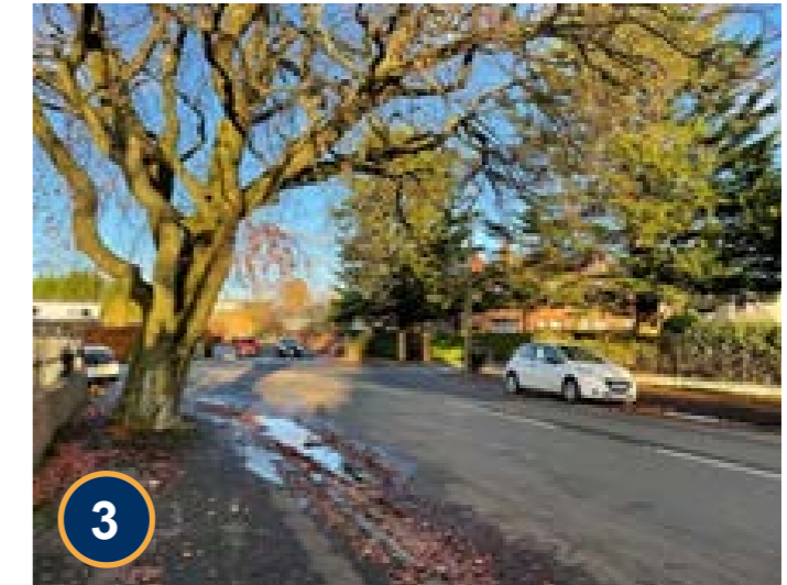
3 Opportunity area on Mansewood Road to facilitate an internal modal filter to address issue of through traffic. Evidence of local flooding which could be addressed using green infrastructure.
