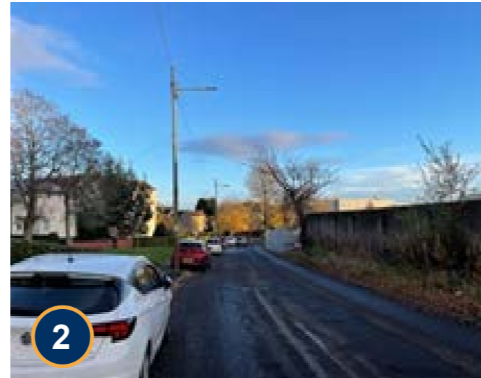
2 Further undesirable footway parking behaviours exhibited on Burnfield Road. Lack of footway on southern side.
