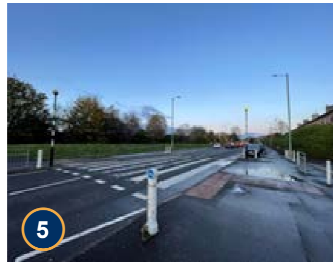
5 Example of existing modal filter at former Auldhouse Road / Holeburn Road junction with pedestrian crossing of Auldhouse Road.
