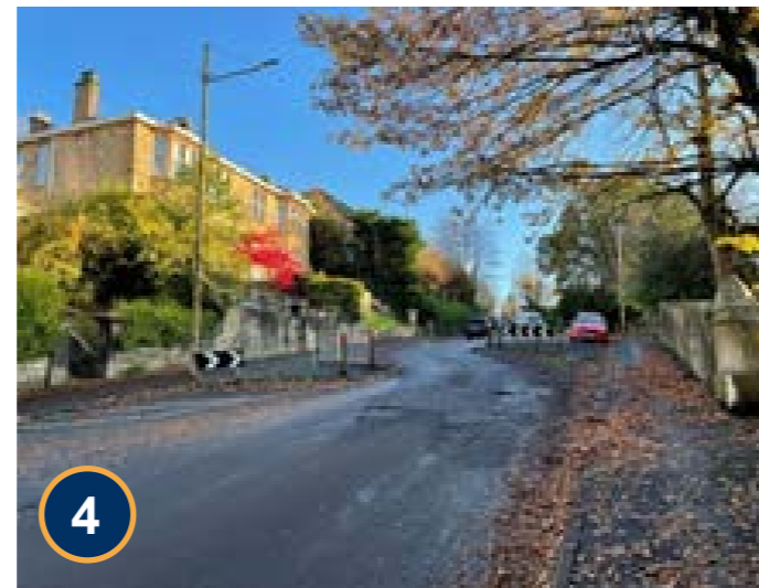
4 Existing traffic calming features on Mansewood Road are over engineered and not very aesthetically pleasing. These appear not to prevent speeding.
